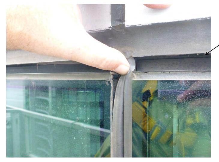
If the ends of the sealant joints are not closed, water is able to infiltrate on top of the primary seal
