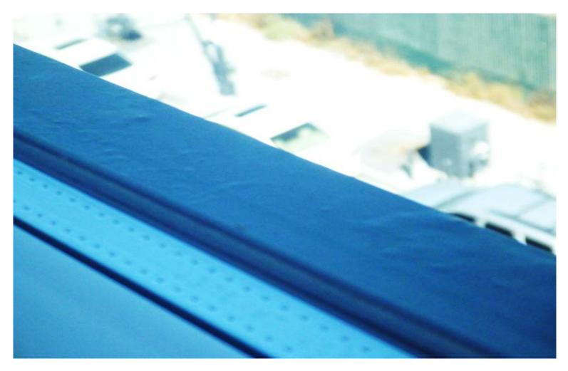
Coating is bubbling on window frames
