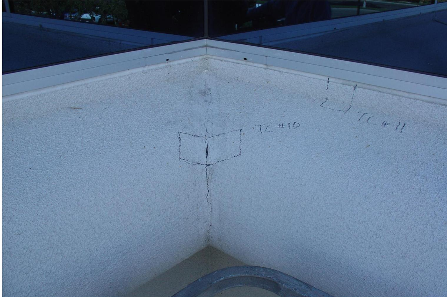
DEFECT: Lack of expansion joint at inside corners
