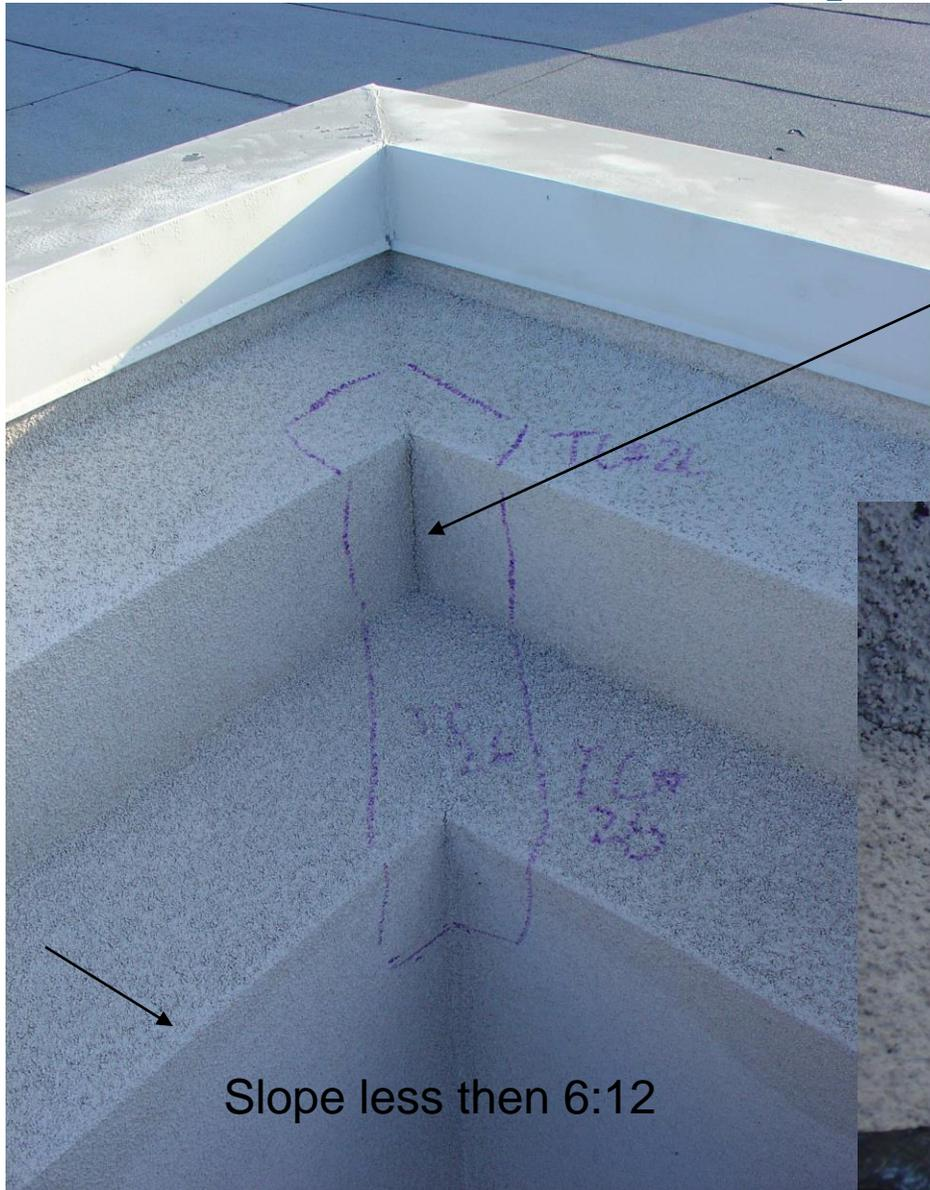
Cracks and splits are caused due to lack for extra reinforcing mesh
