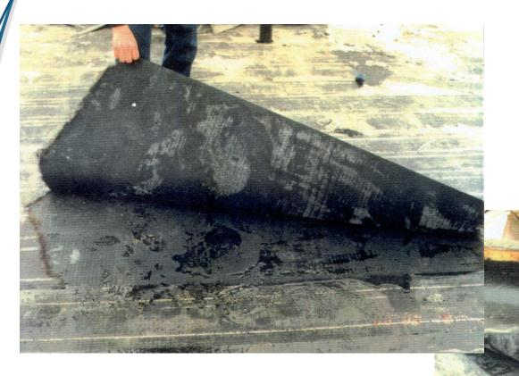
In built up roofs, bitumen is more than just adhesive – it should flow through pores in felt, to form a system.
