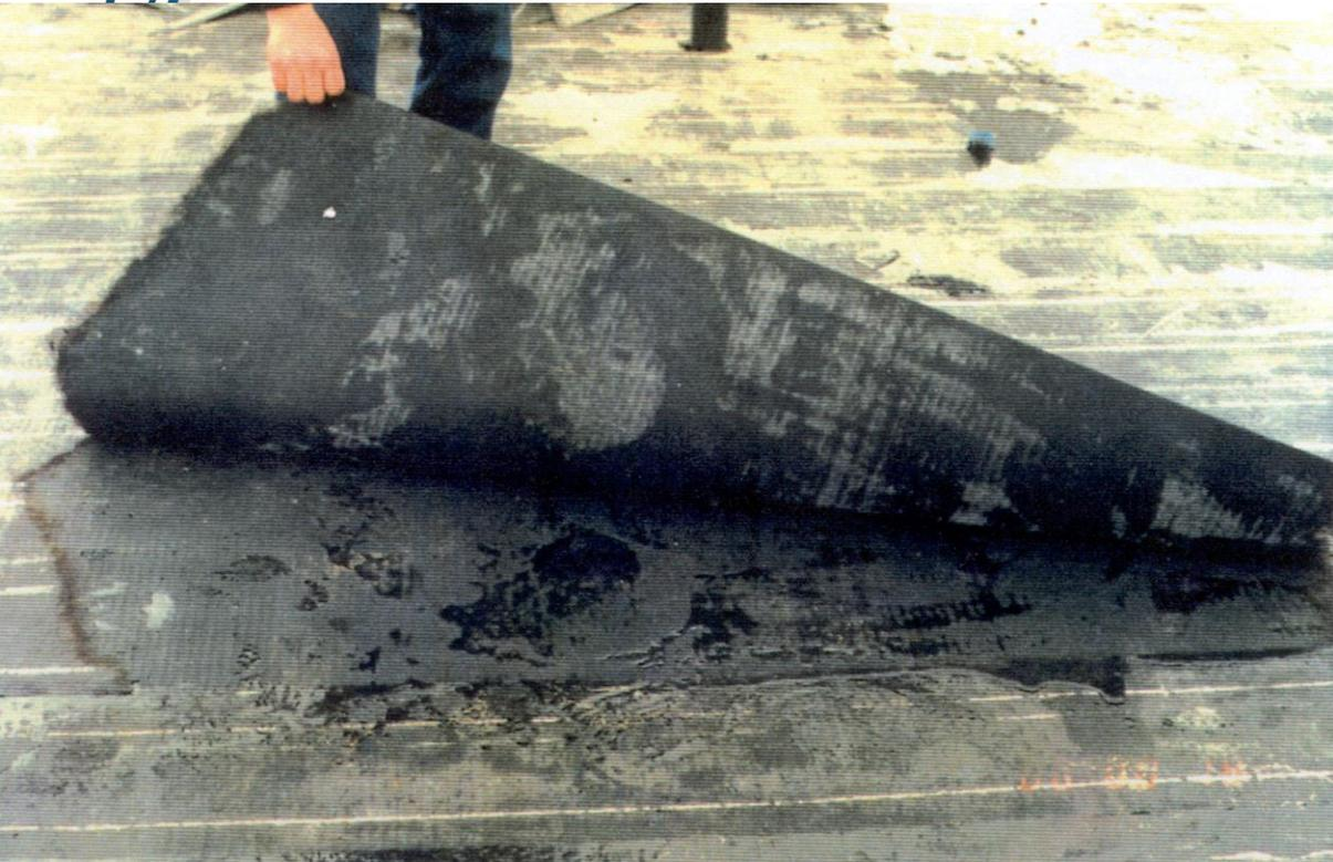
*In built up roofs, bitumen is more than just adhesive – it should flow through pores in felt, to form a system.*
