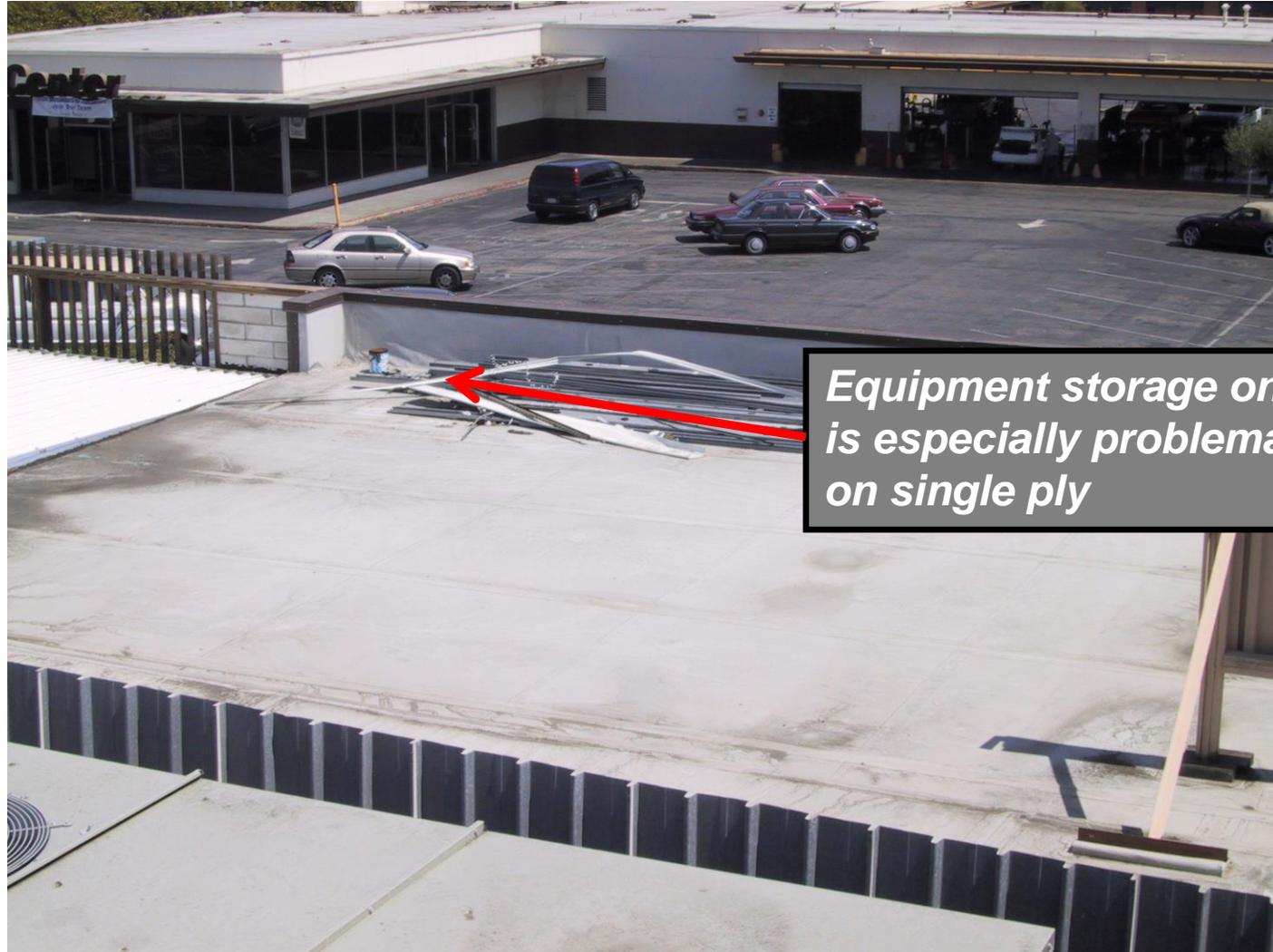
*Equipment storage on roof is especially problematic on single ply*
