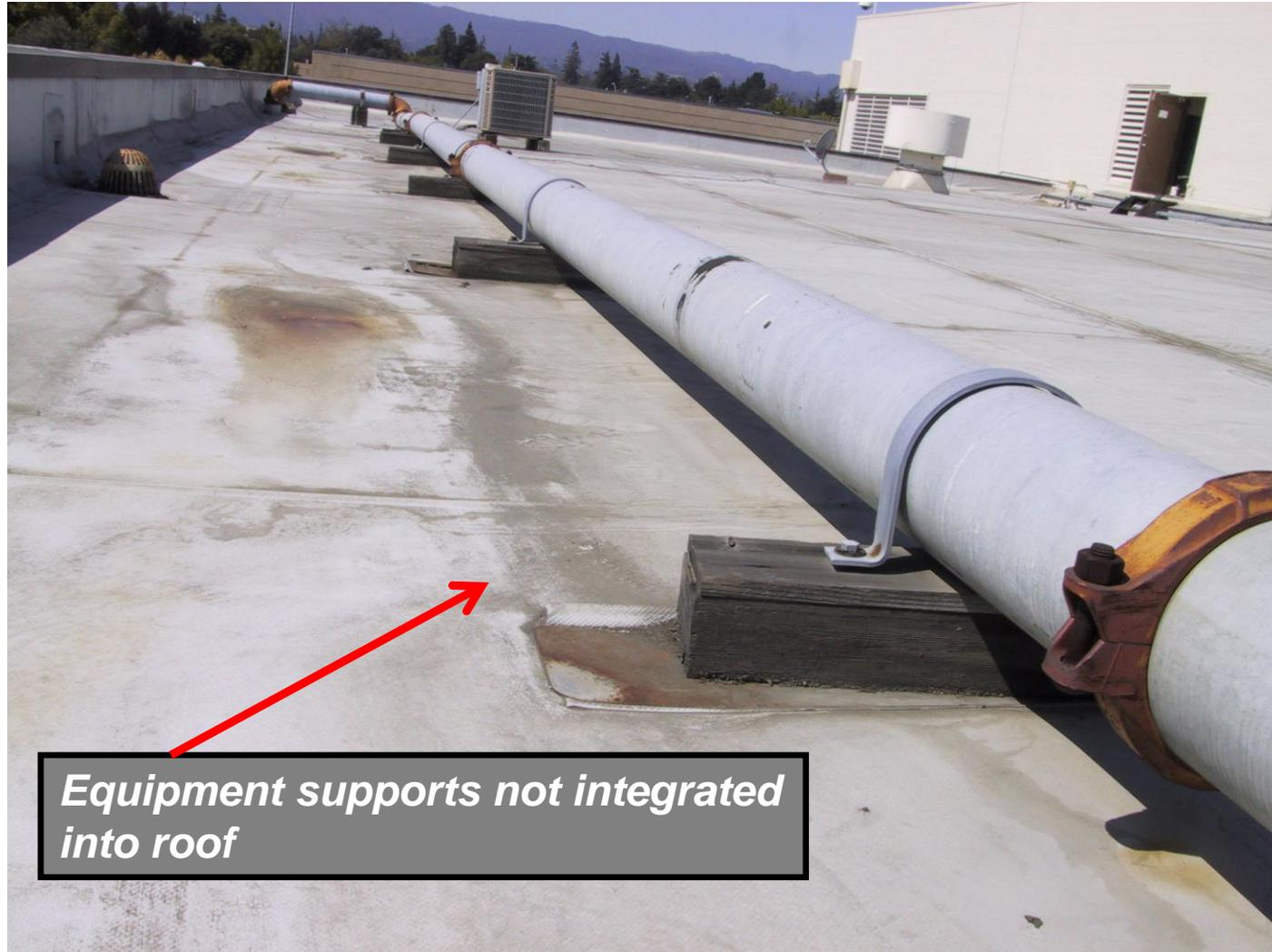
***Equipment supports not integrated into roof***
