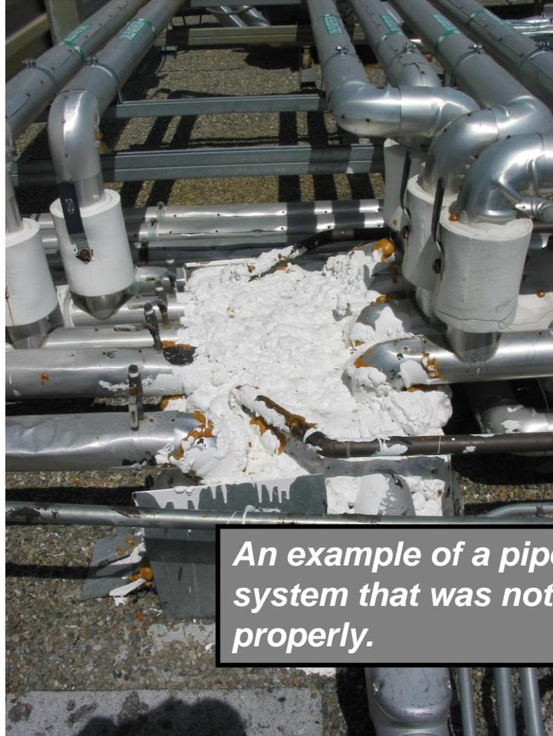
*An example of a pipe penetration system that was not designed properly.*
