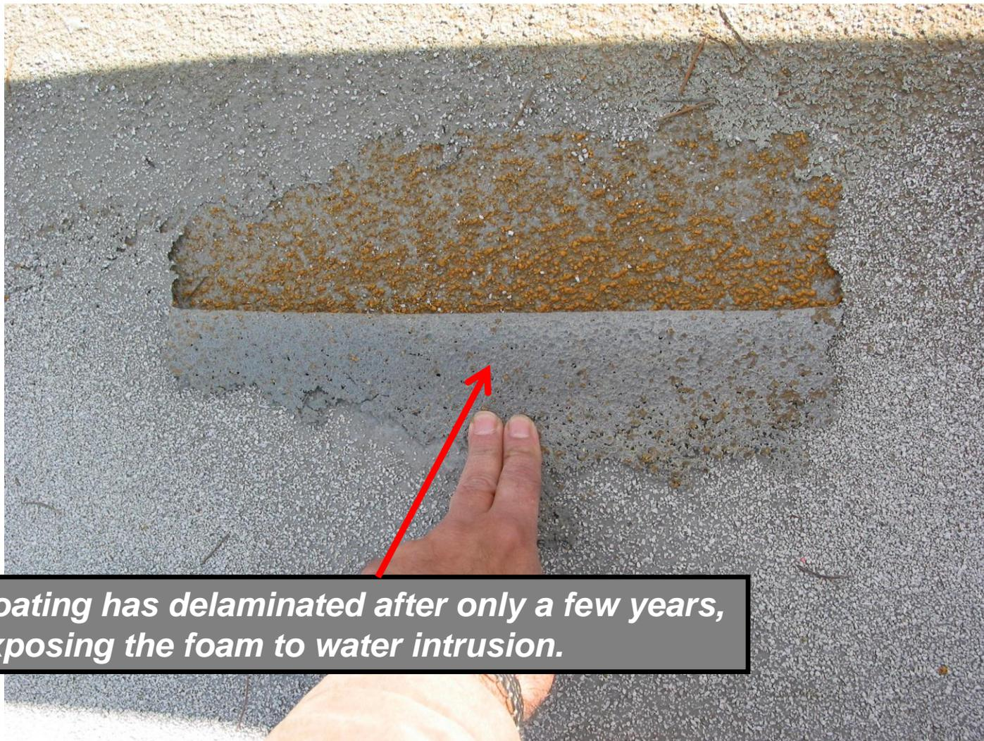
***Coating has delaminated after only a few years, exposing the foam to water intrusion.***
