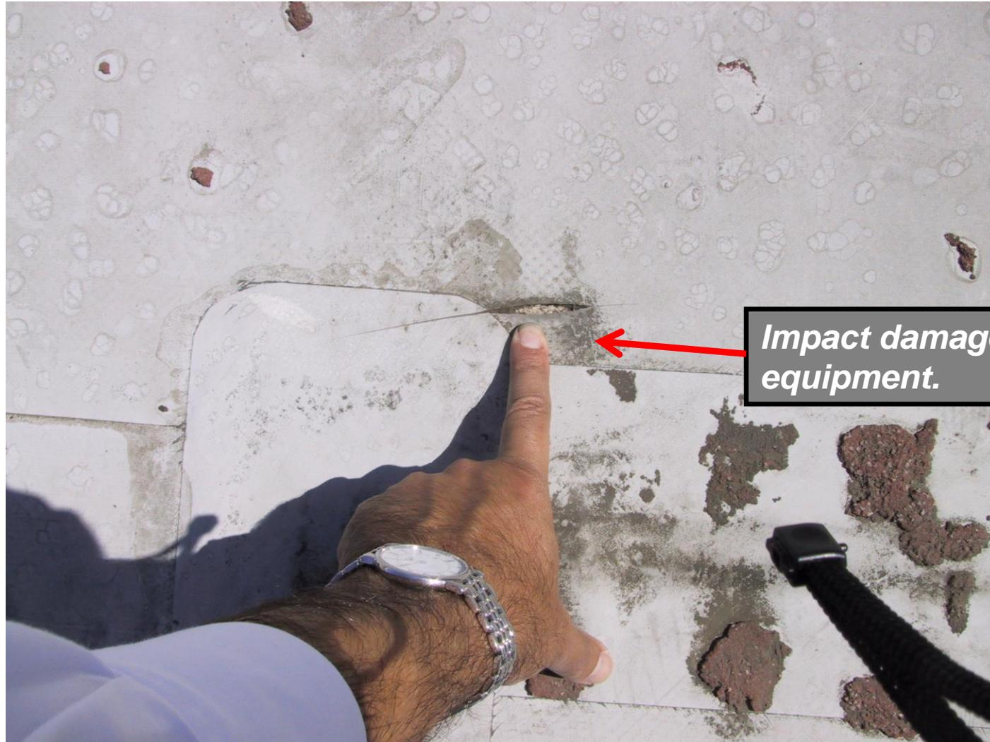
***Impact damage from dropped equipment.***
