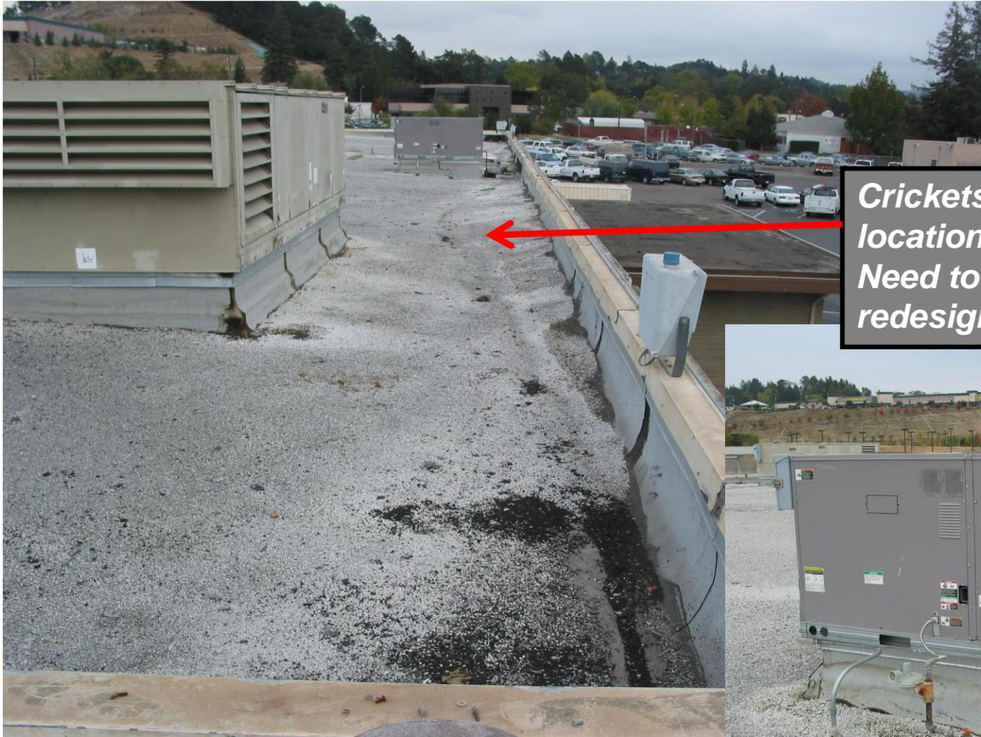
***Cricket is undersized in some locations, or not provided at all. Need to be deeper and redesigned. Note deterioration.***
