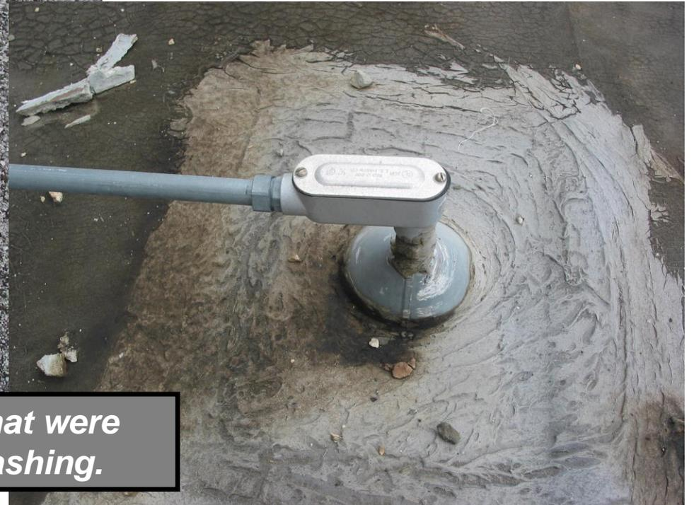
***Two examples of conduits installations that were not designed – installed without proper flashing.***
