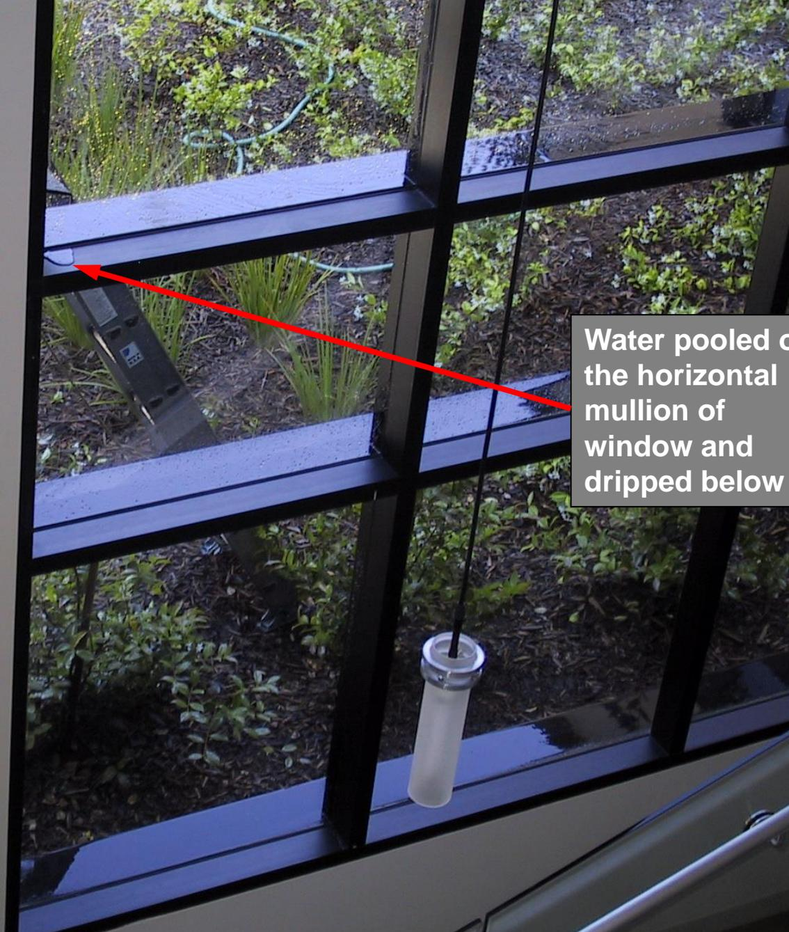
Water pooled on the horizontal mullion of window and dripped below
