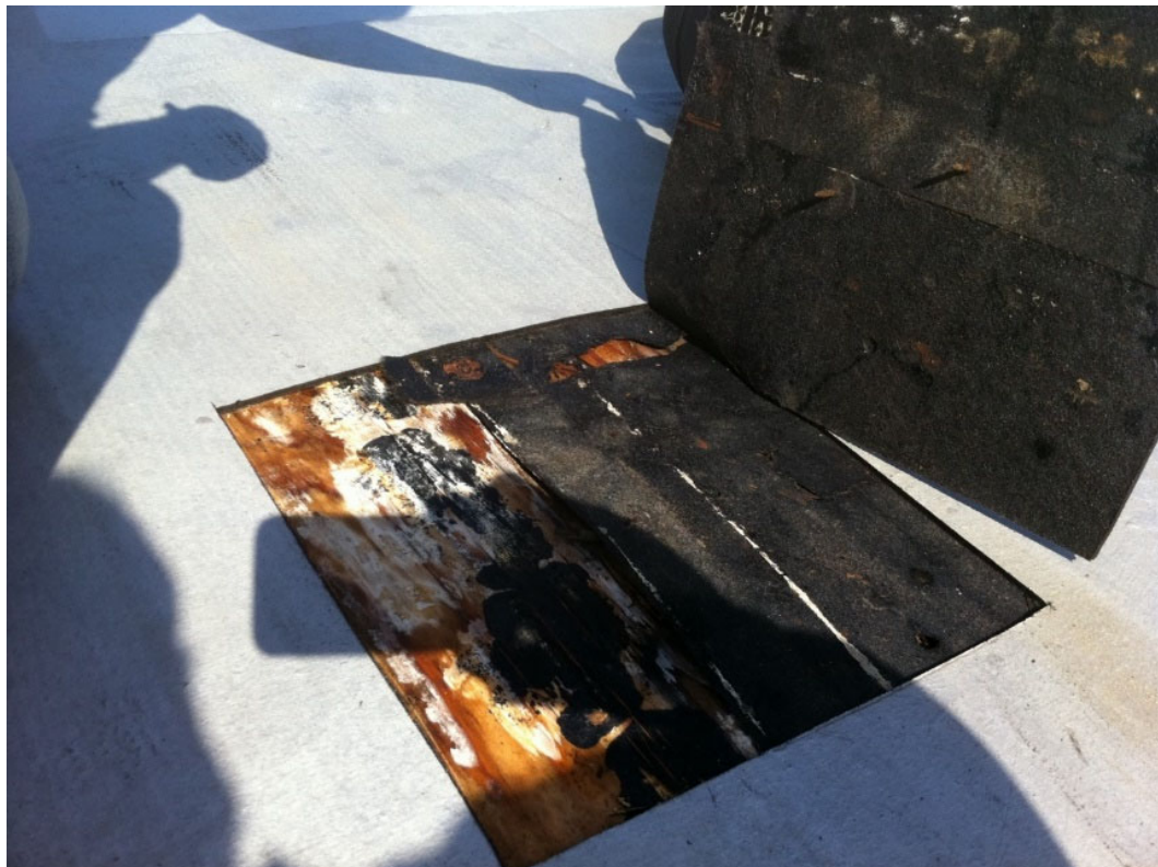
Figure 3: Condensation Damage under a Cool Roof
