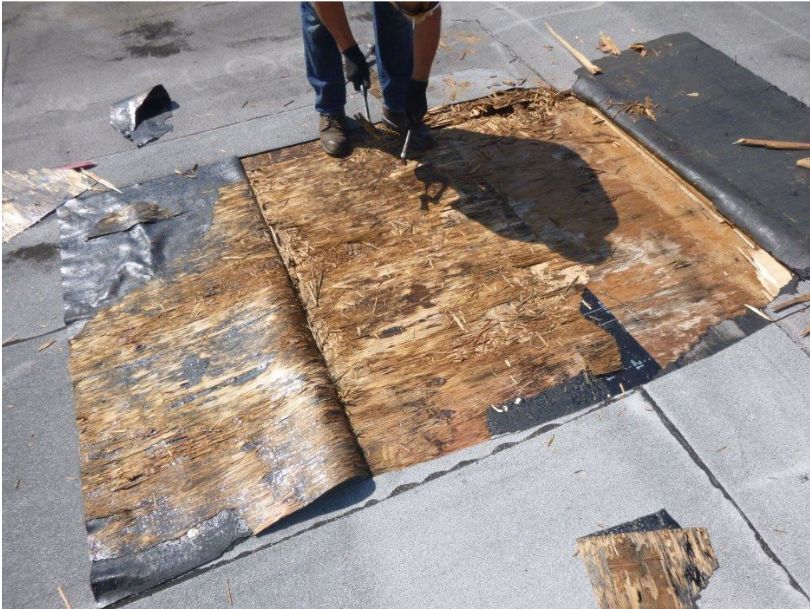
Figure 5: Damage Directly Under Roofing
