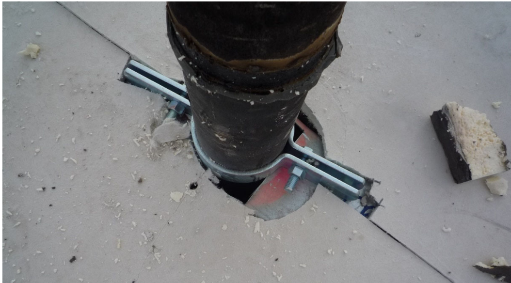
Figure 4: Roof Drains and Other Penetrations Leave Gaps That Can Allow Humid Air to Bypass the Roof Deck
