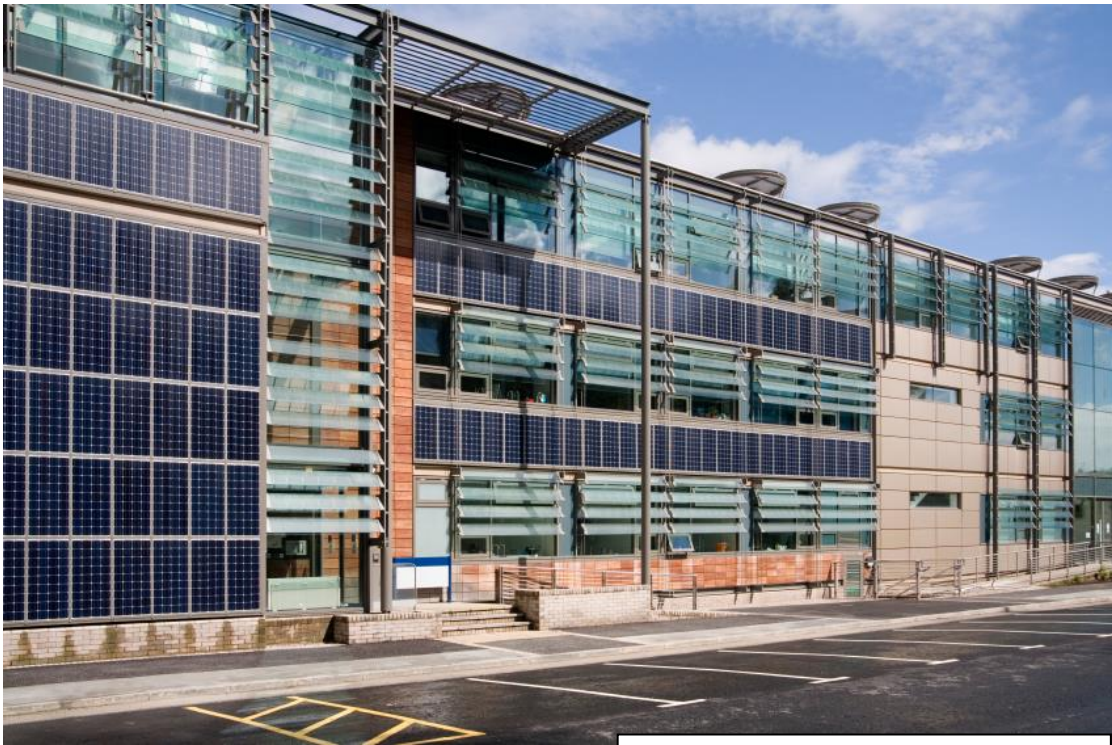
Figure 11. Building integrated PV (BIPV) in a curtain wall.
