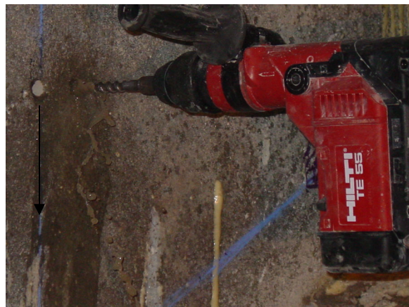
5/8" Zirk Fitting drilling through 18" foundation wall
