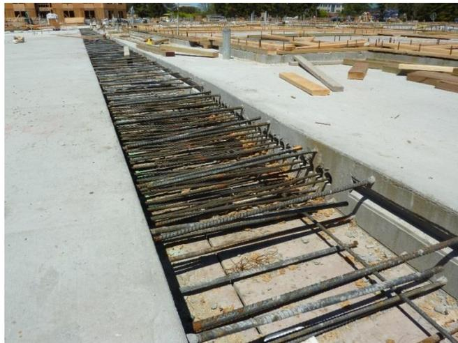
Figure 4: Post-tensioned reinforced concrete slab under construction
