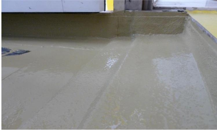
Figure 10: Asphalt modified polyurethane
