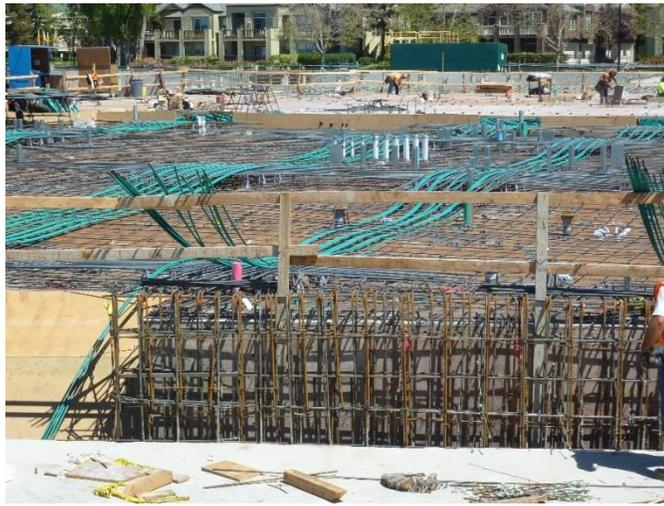
Figure 3: Podium slab with tensioning cables and reinforcing steel
