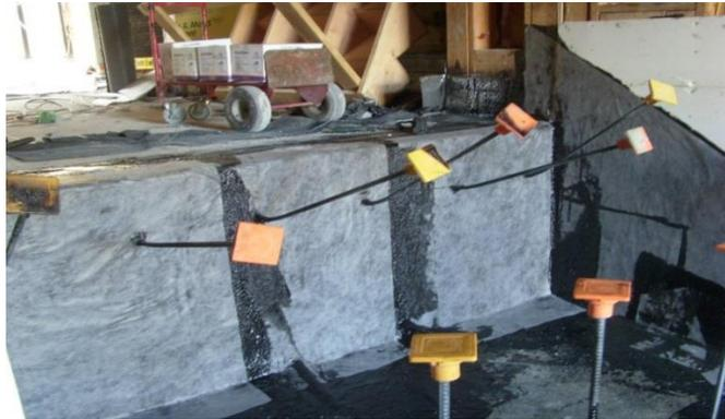
Figure 14: Waterproofing around reinforcing steel
