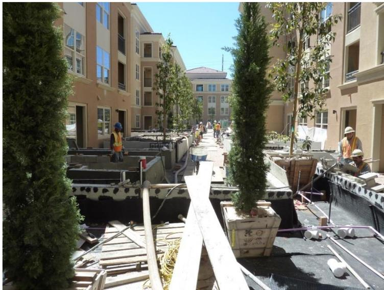
Figure 2: Typical Podium under construction with waterproofing complete inside of planters. Due to the heavy construction traffic, waterproofing membrane is phased and installed last, before the wearing course.
