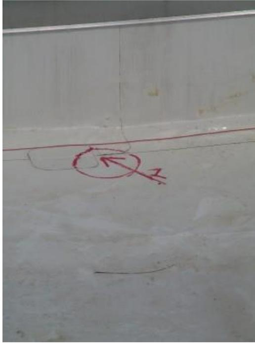
Figure 19: Pinhole leak discovered using EFVM
