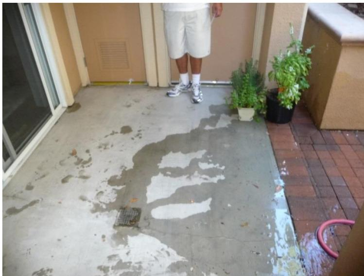
Figure 21: Water flows from the door even though it never flows to it
