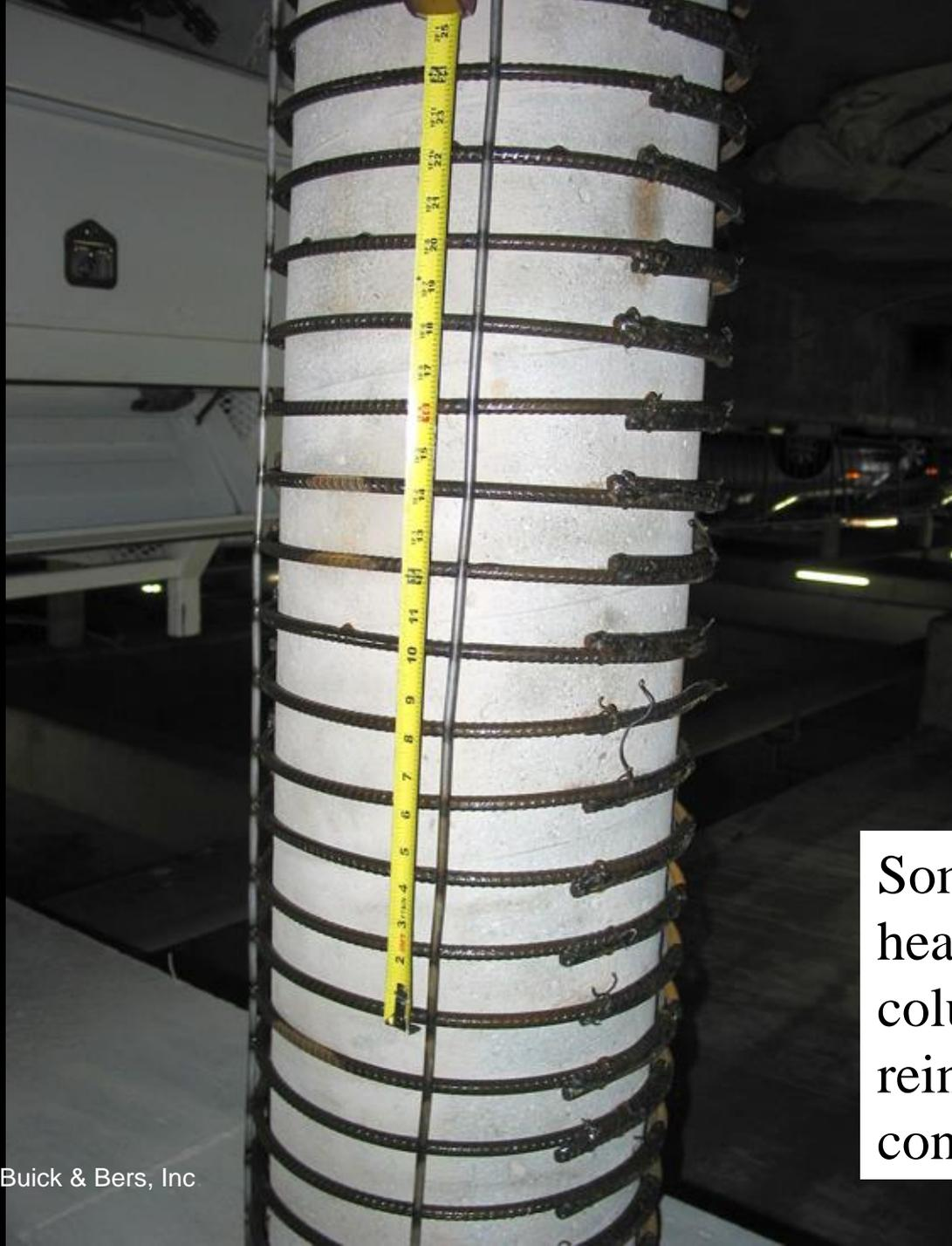
Some of the heavily stressed columns were reinforced with concrete and rebar
