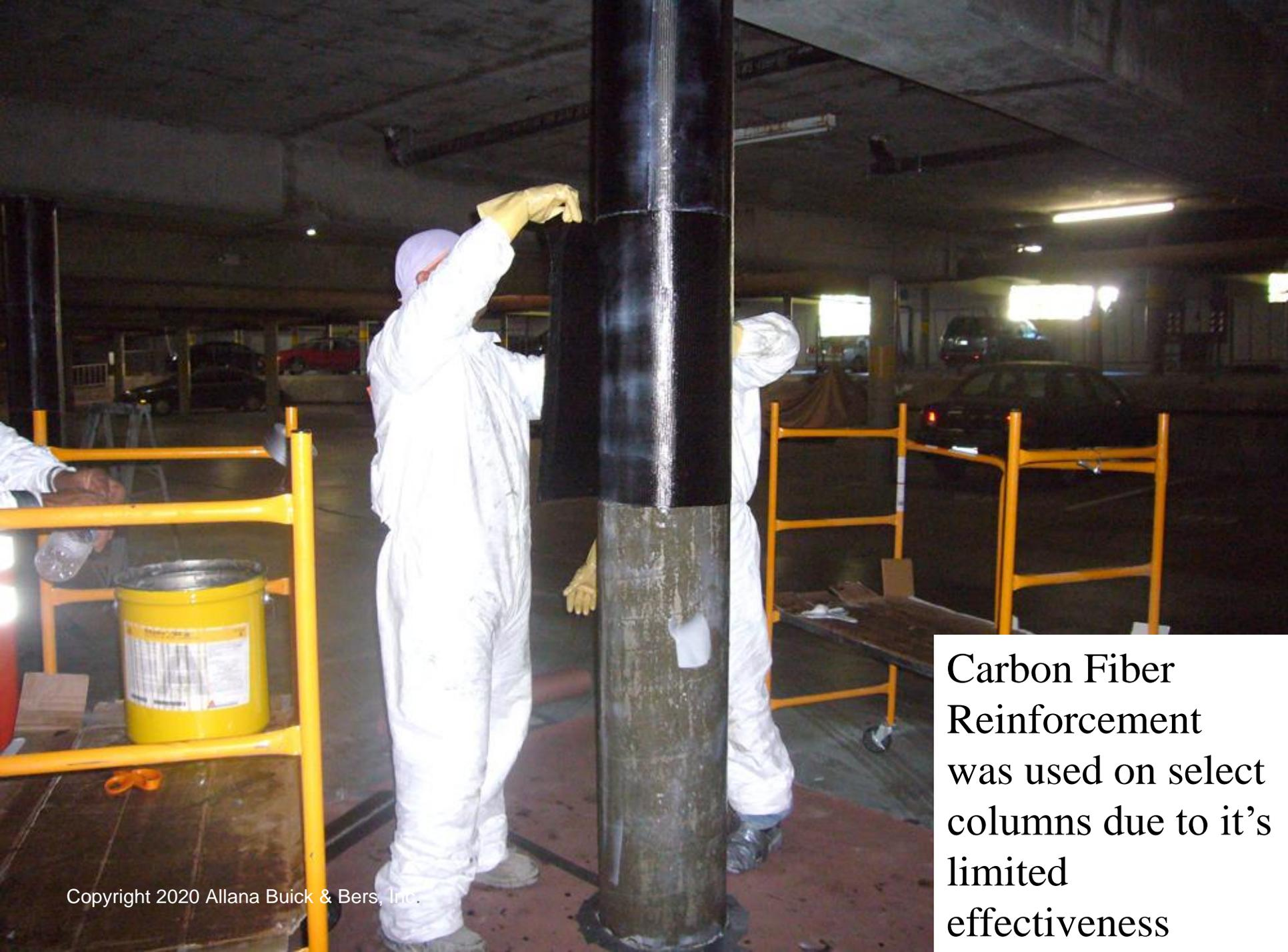
Carbon Fiber Reinforcement was used on select columns due to it's limited effectiveness
