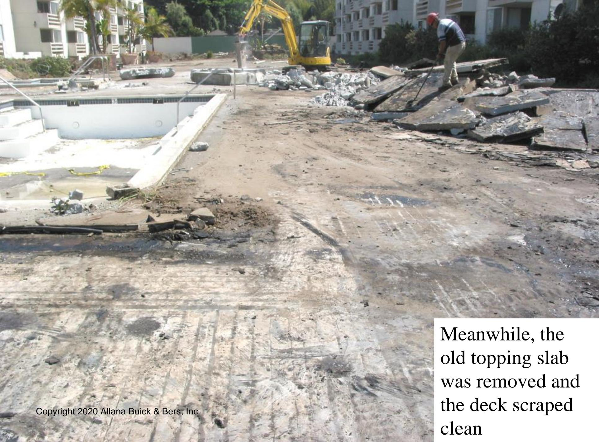
Meanwhile, the old topping slab was removed and the deck scraped clean
