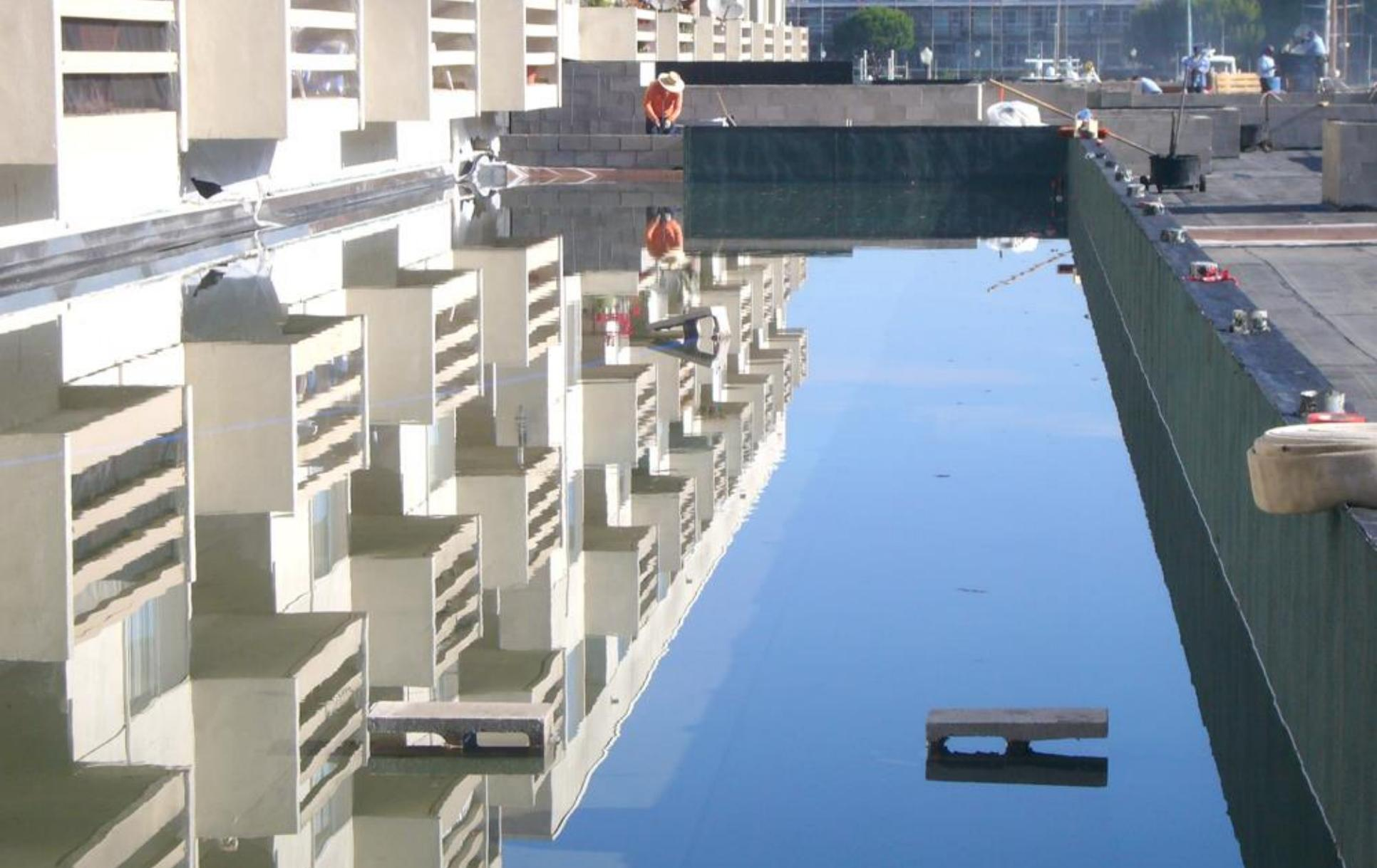
Sections of the Deck were water tested prior to being filled
