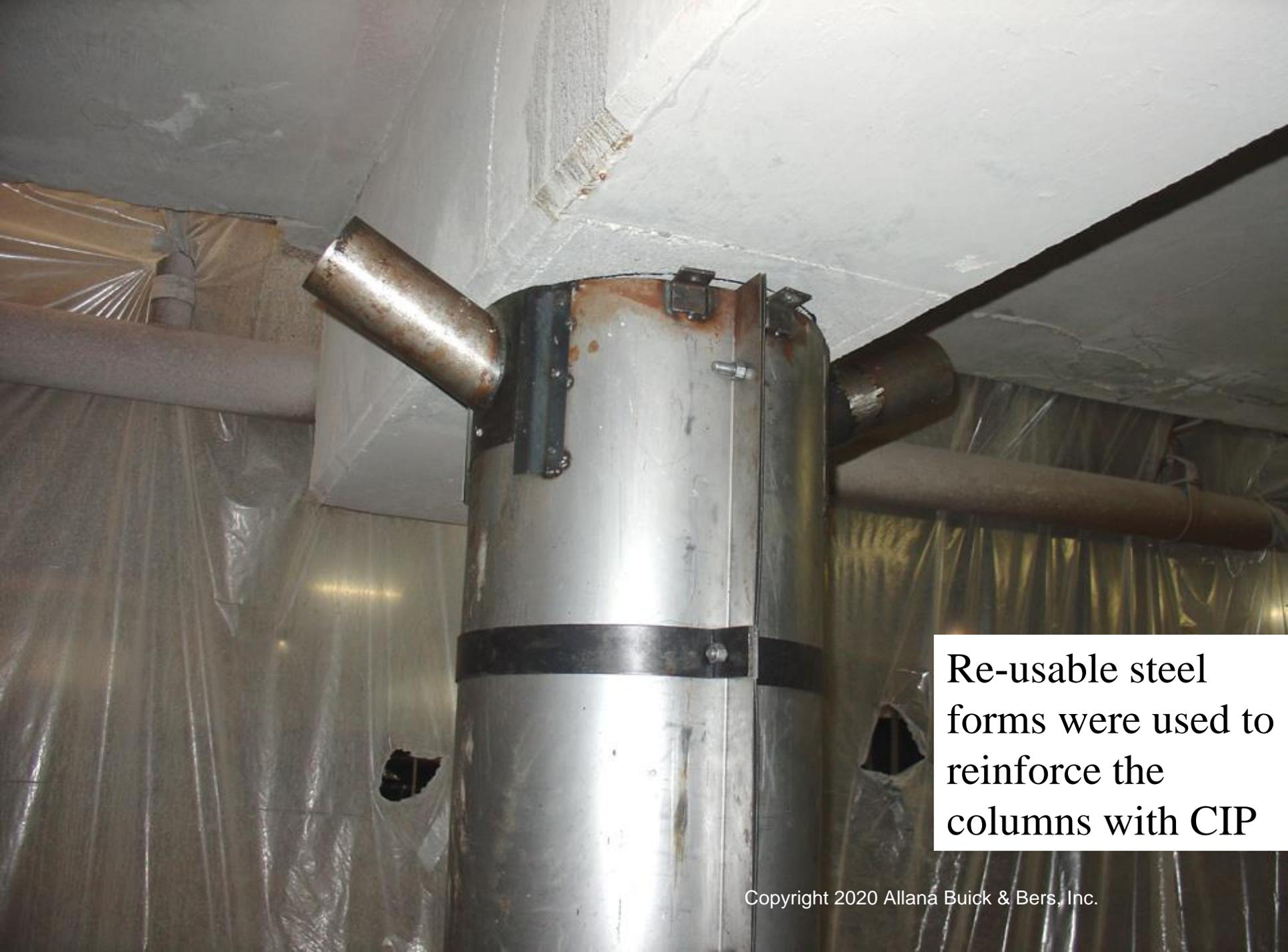
Re-usable steel forms were used to reinforce the columns with CIP
