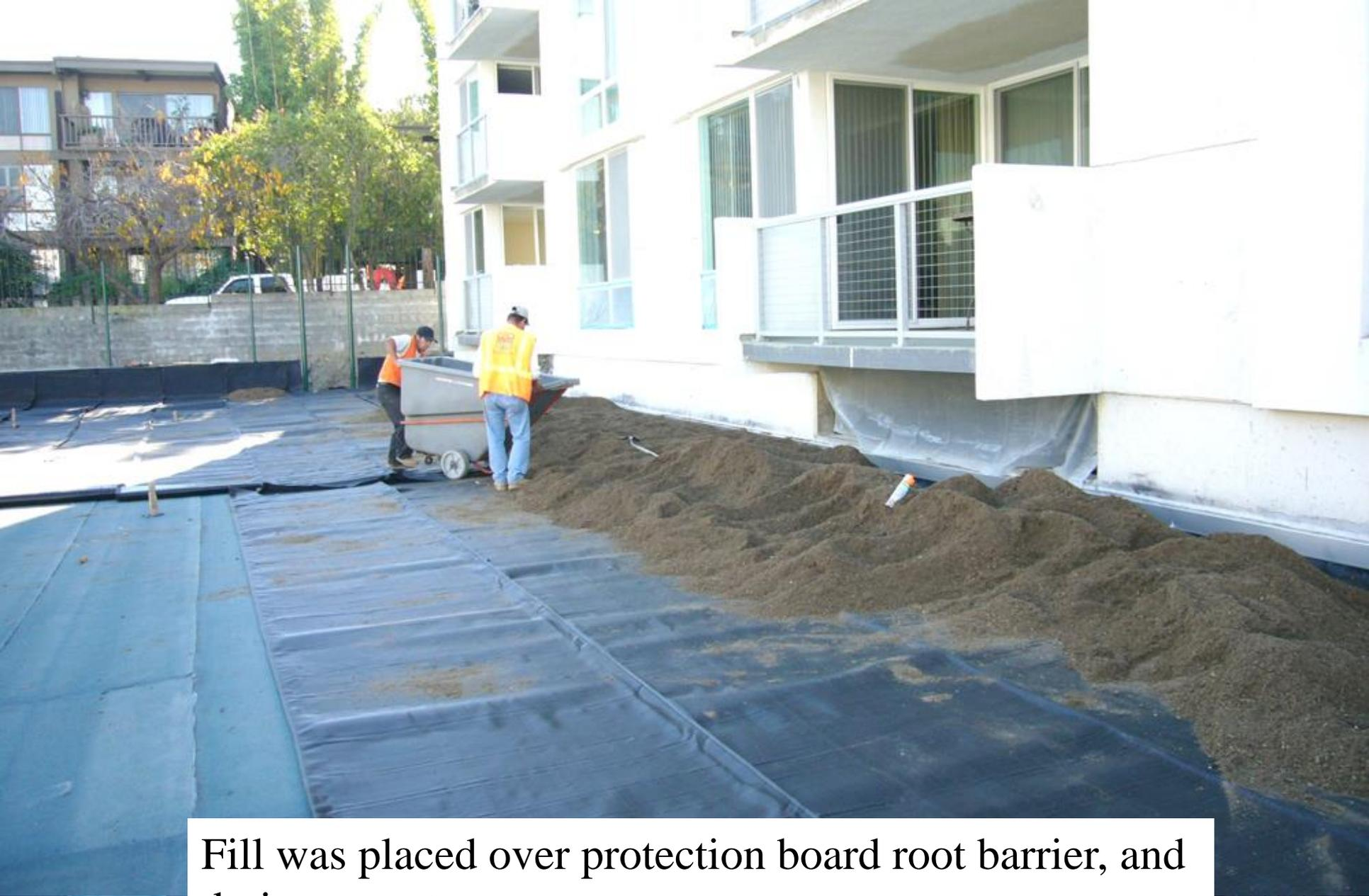
Fill was placed over protection board root barrier, and drainage mat
