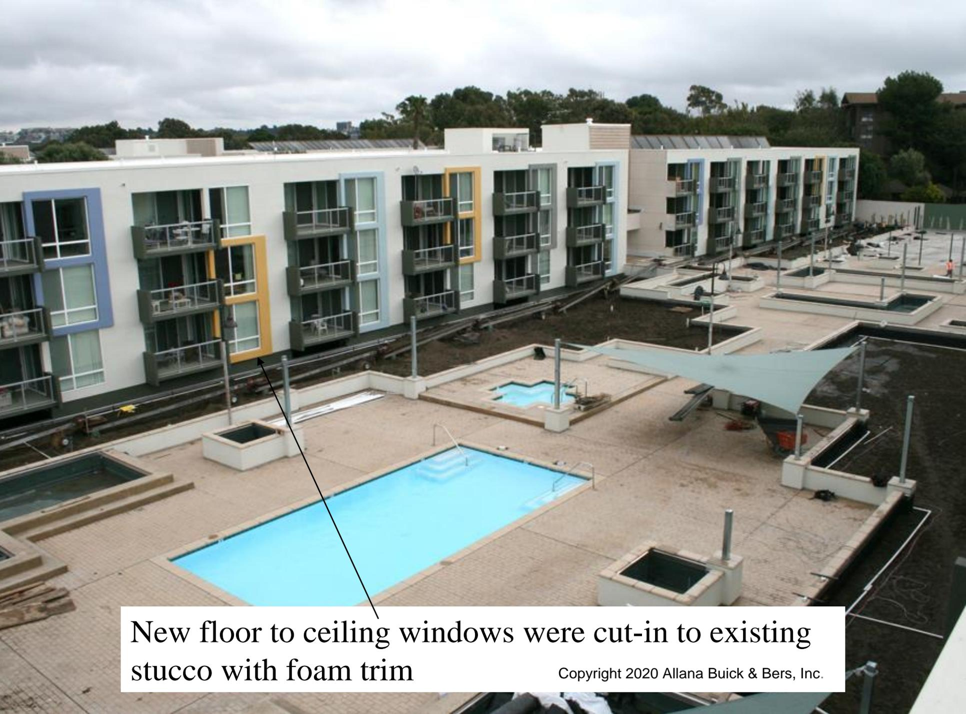
New floor to ceiling windows were cut-in to existing stucco with foam trim
