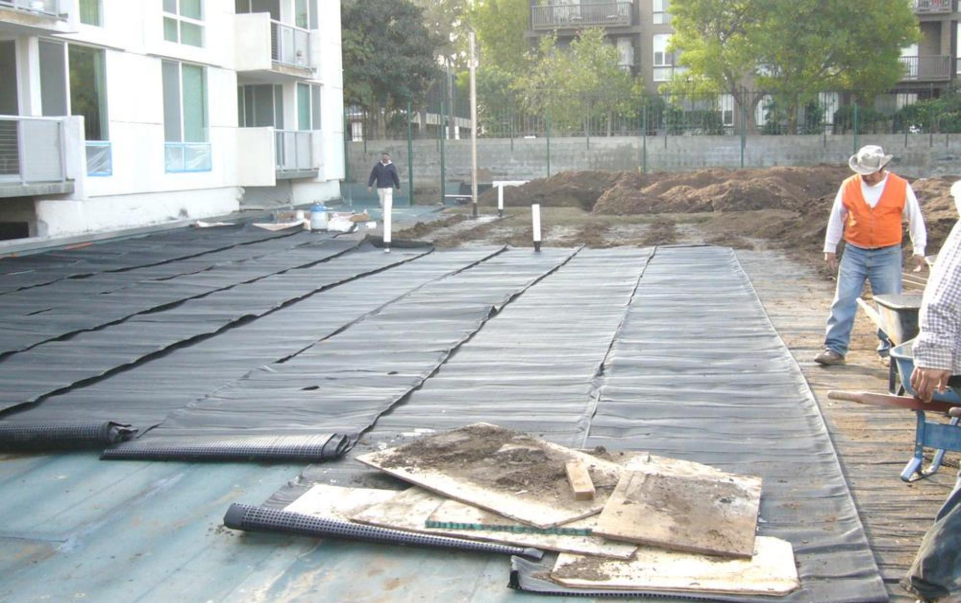
Fill was placed over protection board root barrier, and drainage mat
