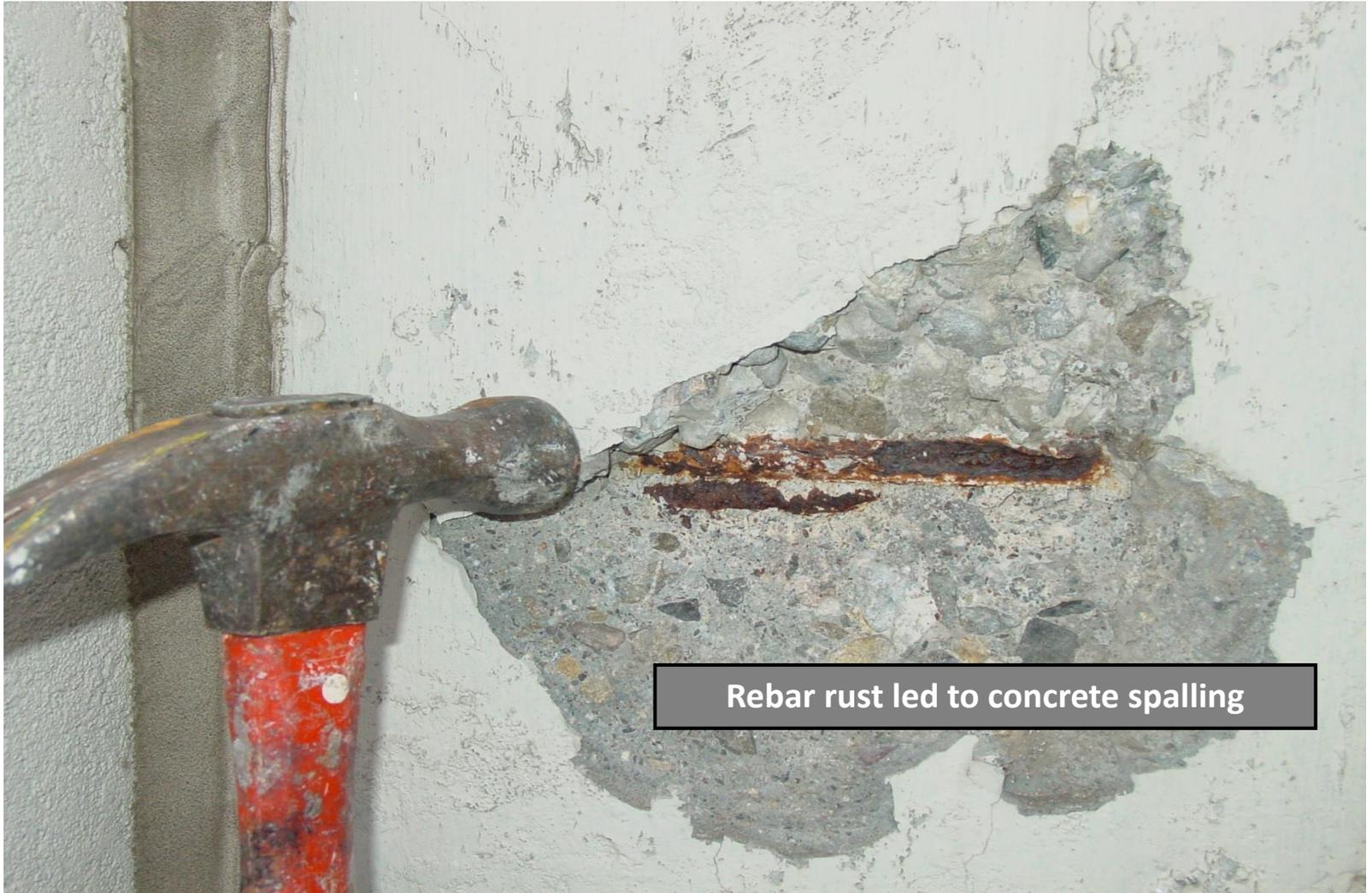
Rebar rust led to concrete spalling
