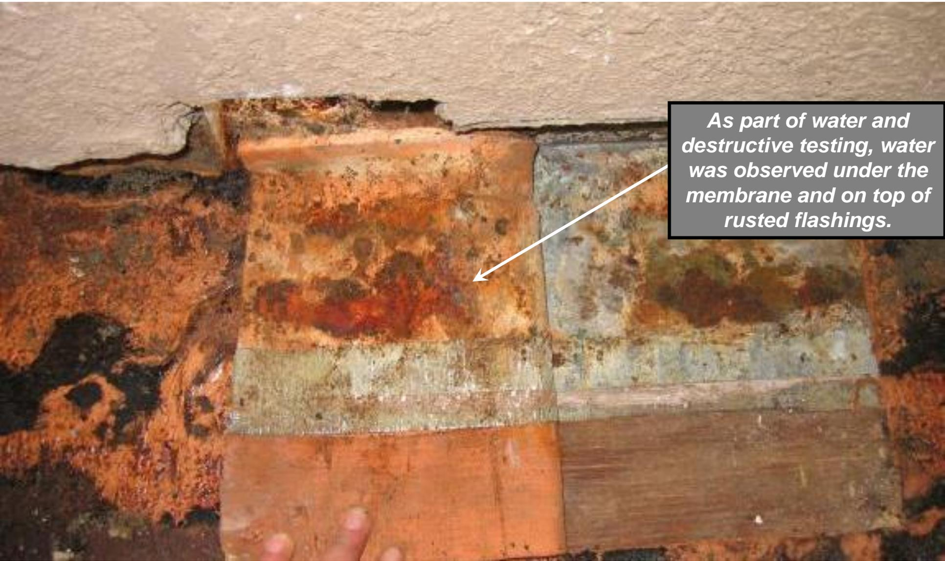
*As part of water and destructive testing, water was observed under the membrane and on top of rusted flashings.*
