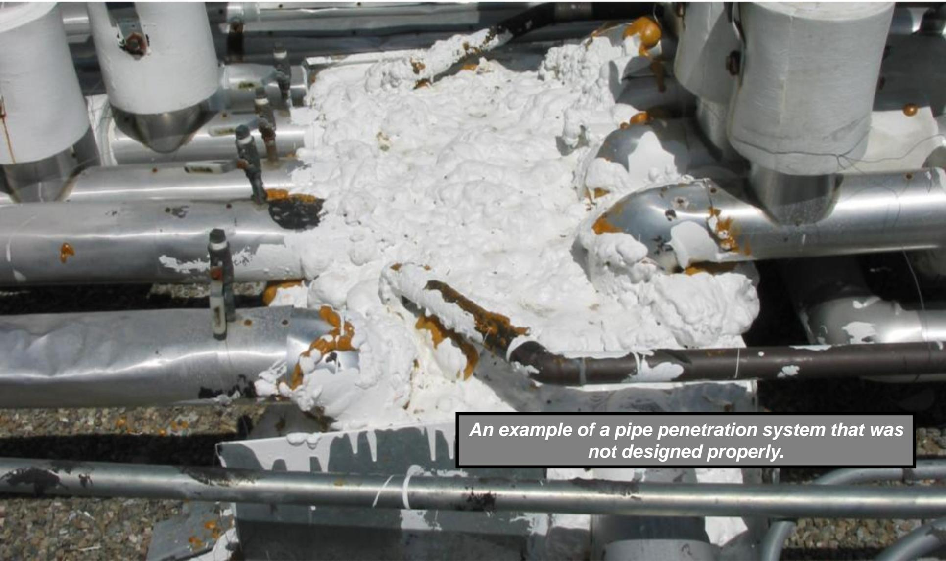
*An example of a pipe penetration system that was not designed properly.*
