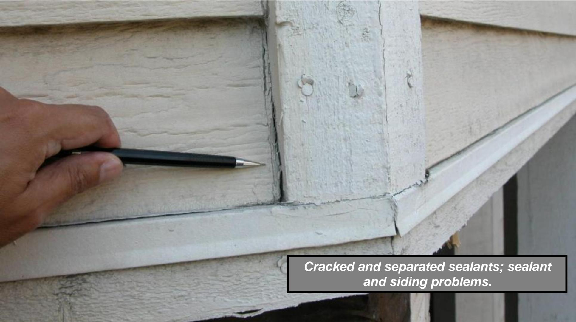
*Cracked and separated sealants; sealant and siding problems.*
