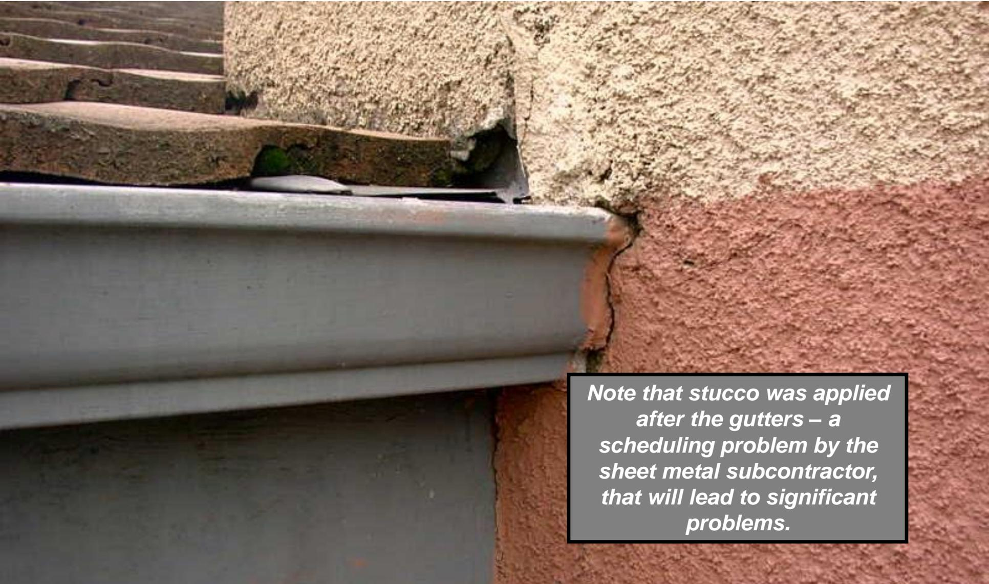
*Note that stucco was applied after the gutters – a scheduling problem by the sheet metal subcontractor, that will lead to significant problems.*
