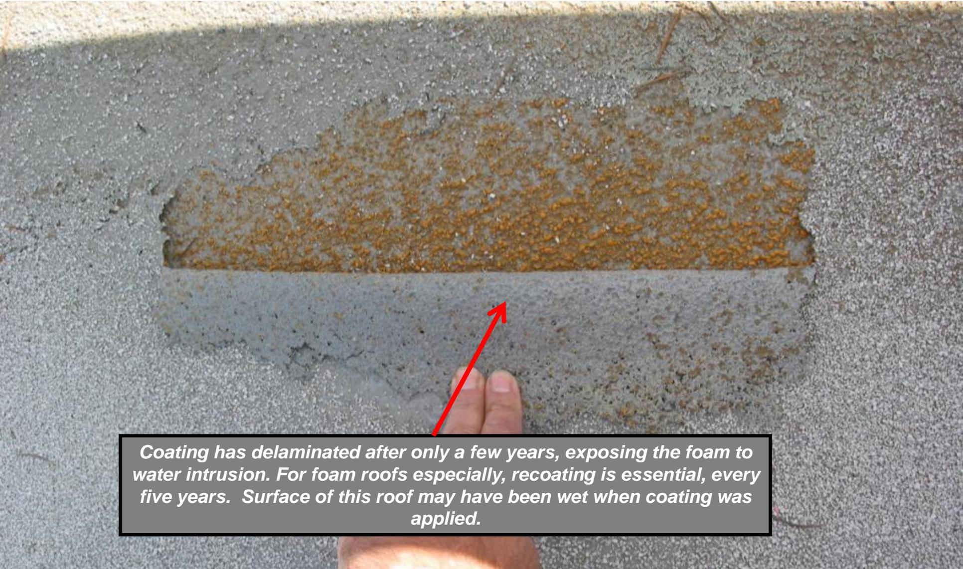
*Coating has delaminated after only a few years, exposing the foam to water intrusion. For foam roofs especially, recoating is essential, every five years. Surface of this roof may have been wet when coating was applied.*
