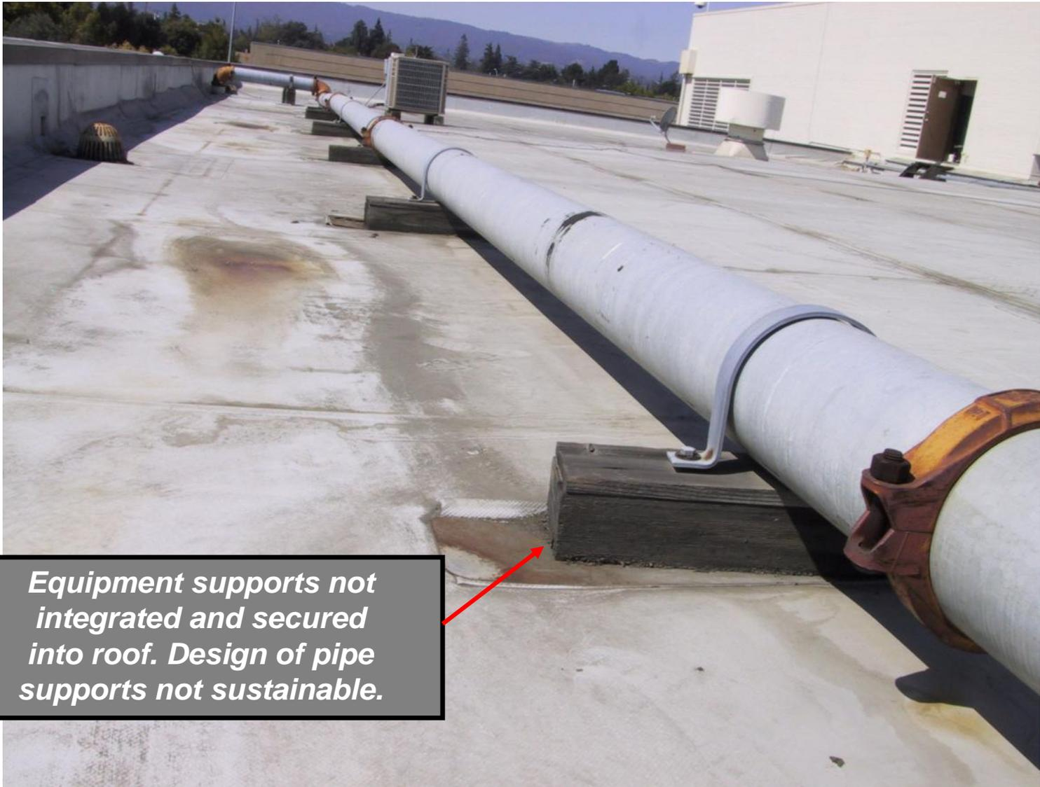
*Equipment supports not integrated and secured into roof. Design of pipe supports not sustainable.*
