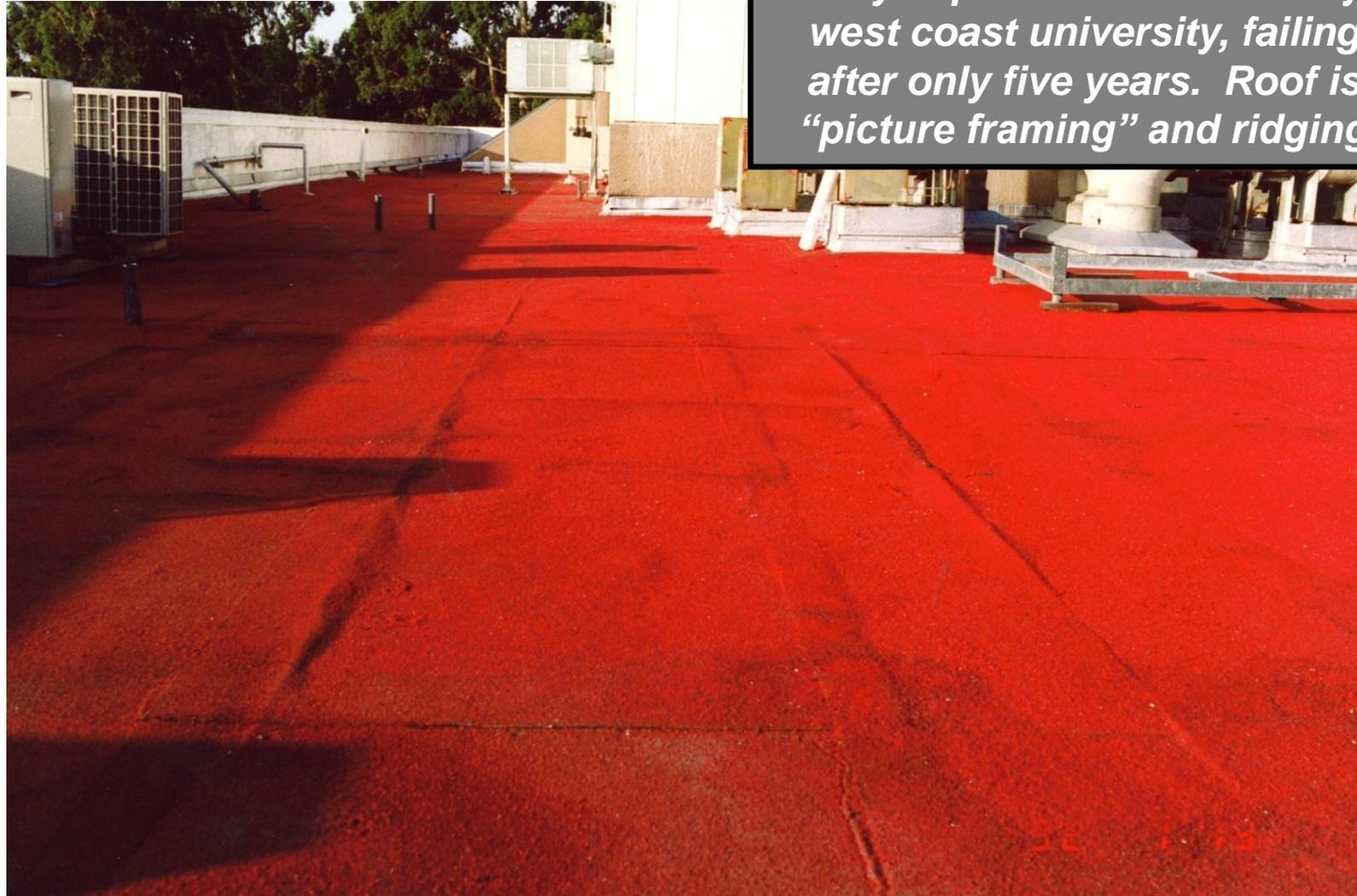
***DEFECT: Improper securement of roof. Inappropriate insulation fasteners, poorly installed, causing cupping of insulation material.***
