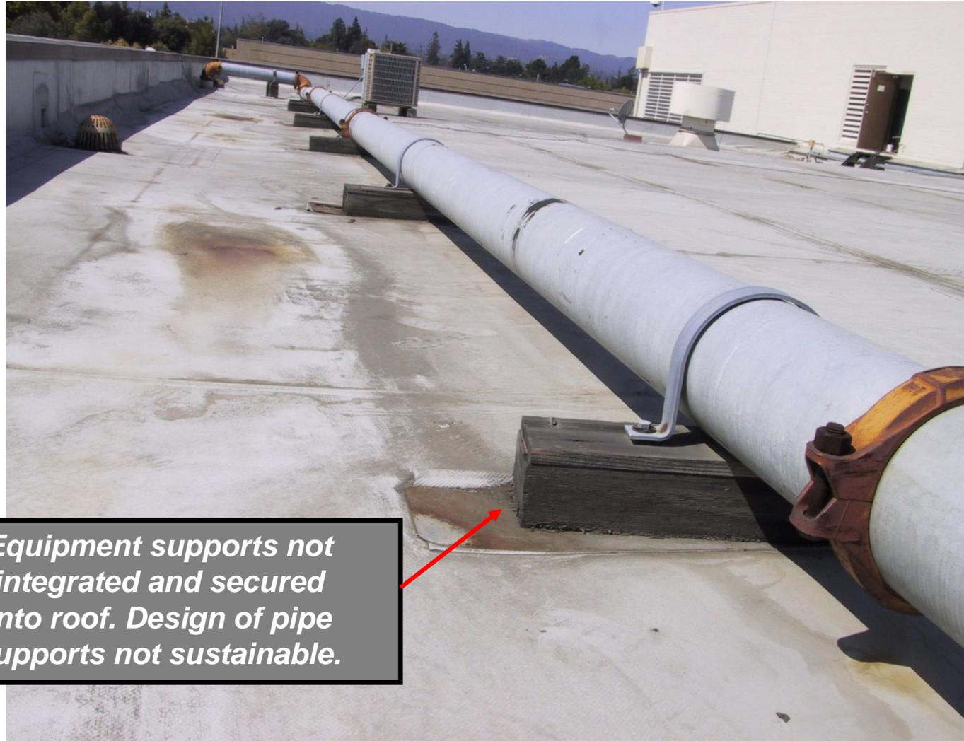
*Equipment supports not integrated and secured into roof. Design of pipe supports not sustainable.*
