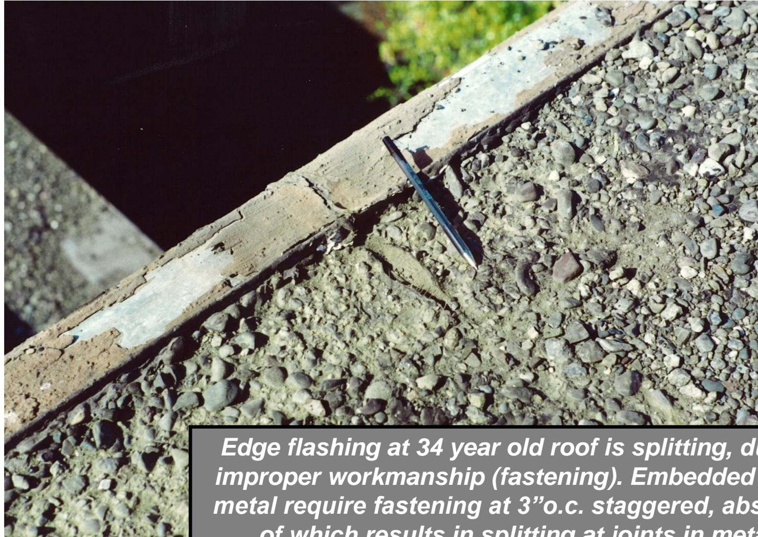
*Edge flashing at 34 year old roof is splitting, due to improper workmanship (fastening). Embedded edge metal require fastening at 3"o.c. staggered, absence of which results in splitting at joints in metal*
