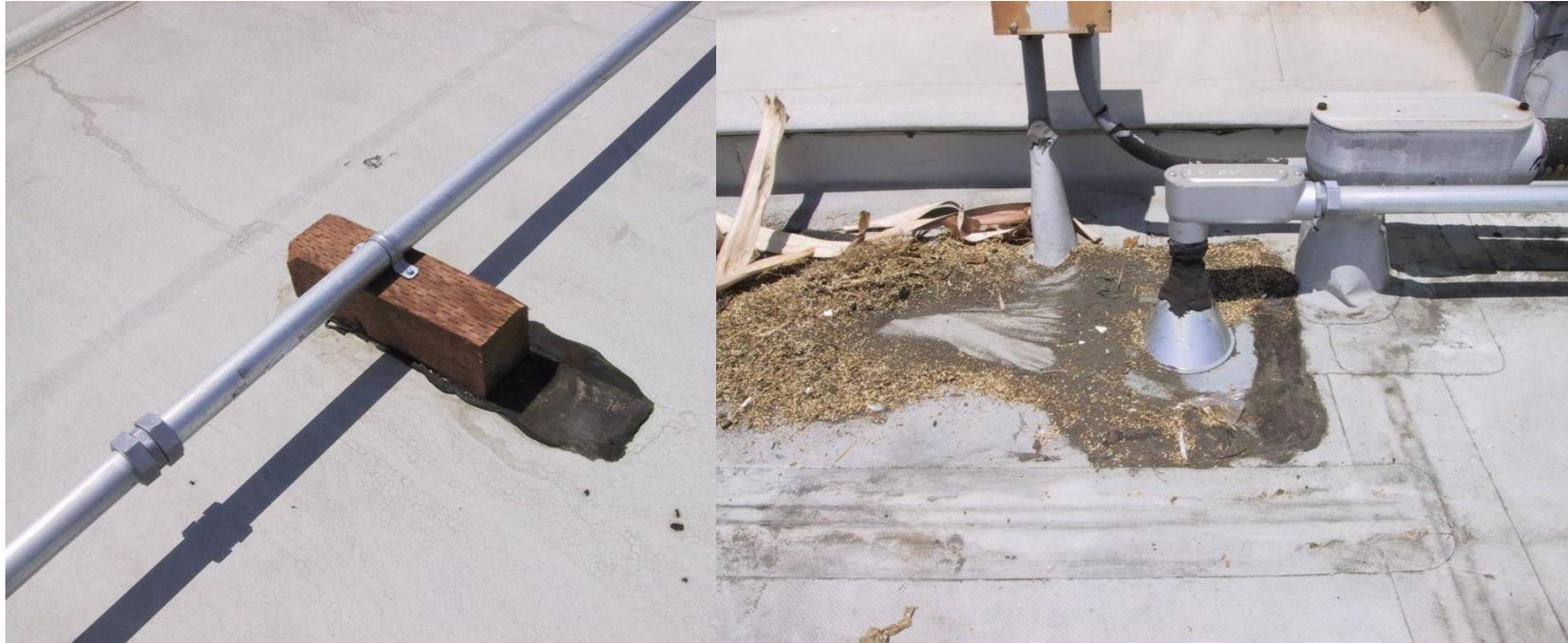
**New electrical pipe added, pipe jack set in mastic (not properly flashed with single ply) and wood block set in mastic (incompatible with PVC).**
