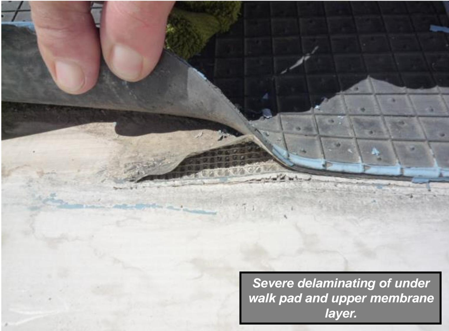
*Severe delaminating of under walk pad and upper membrane layer.*
