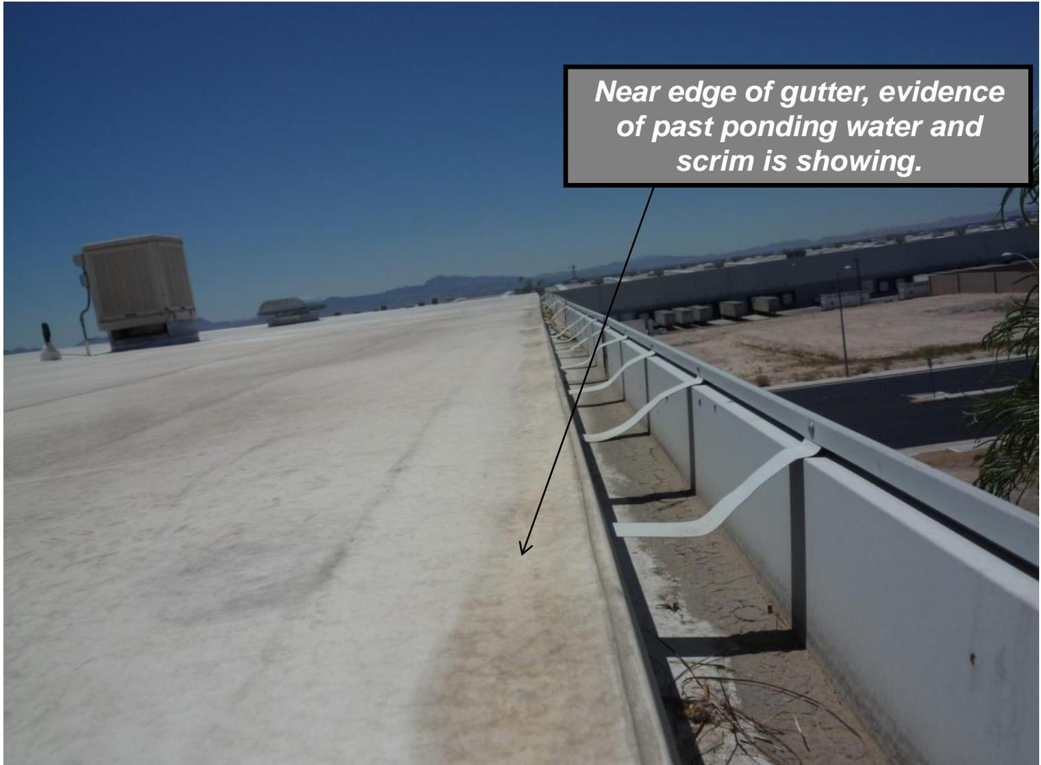
*Near edge of gutter, evidence of past ponding water and scrim is showing.*
