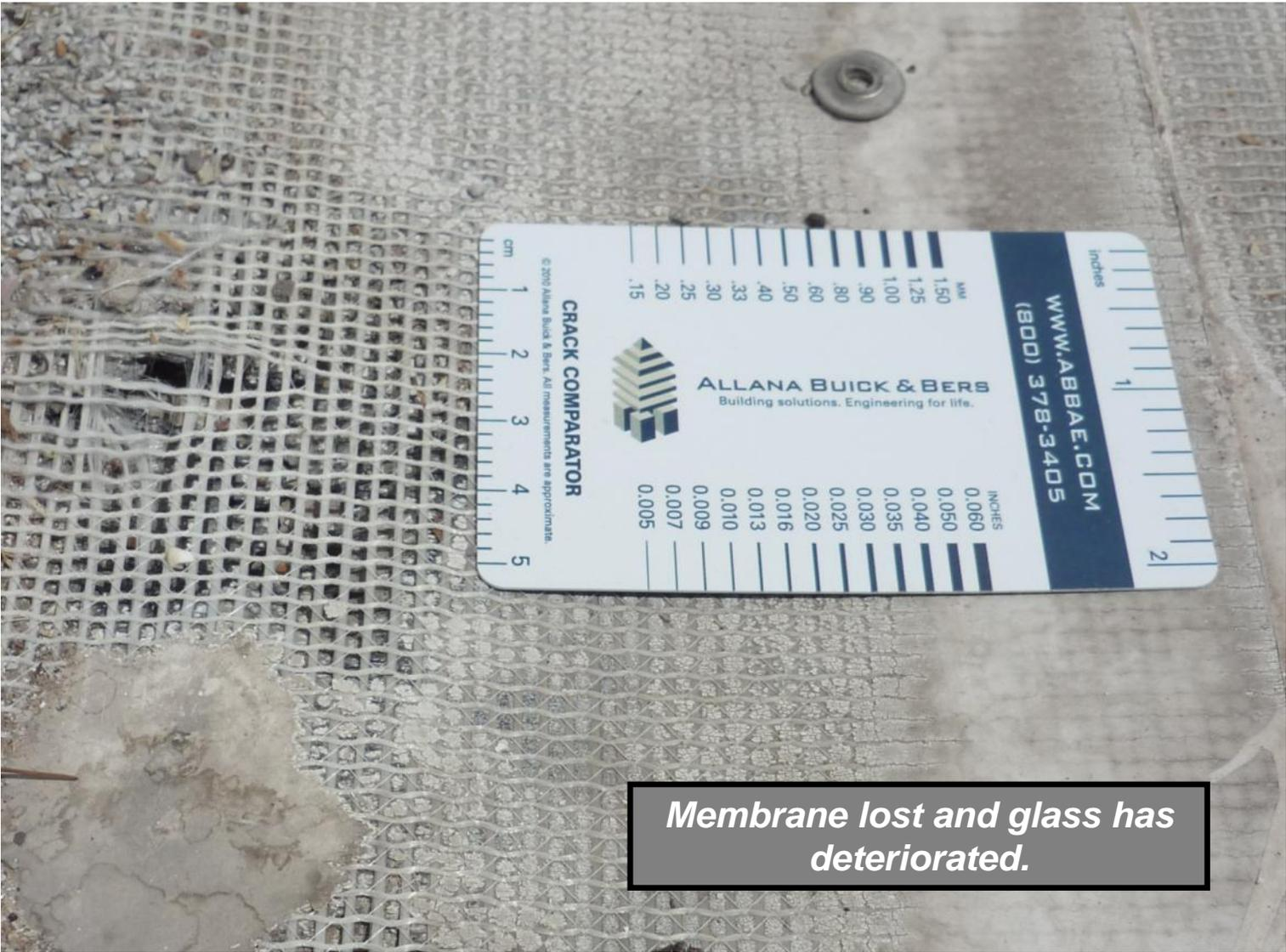
*Membrane lost and glass has deteriorated.*
