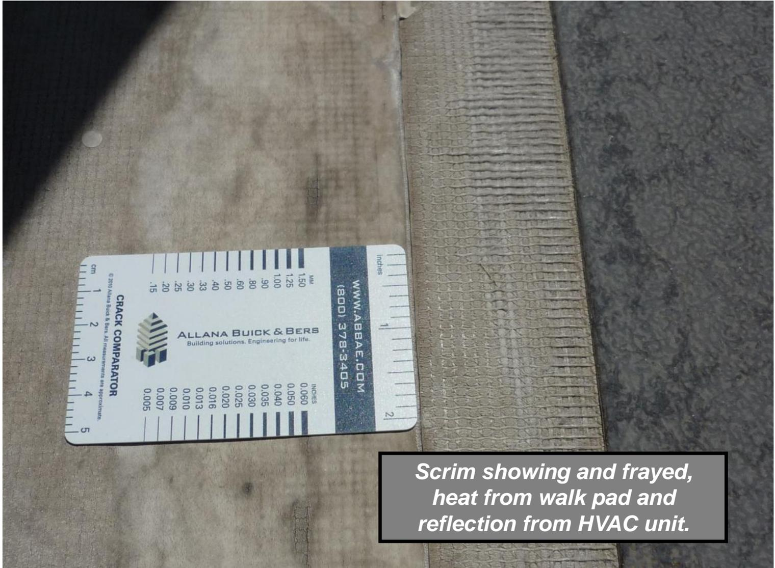
*Scrim showing and frayed, heat from walk pad and reflection from HVAC unit.*
