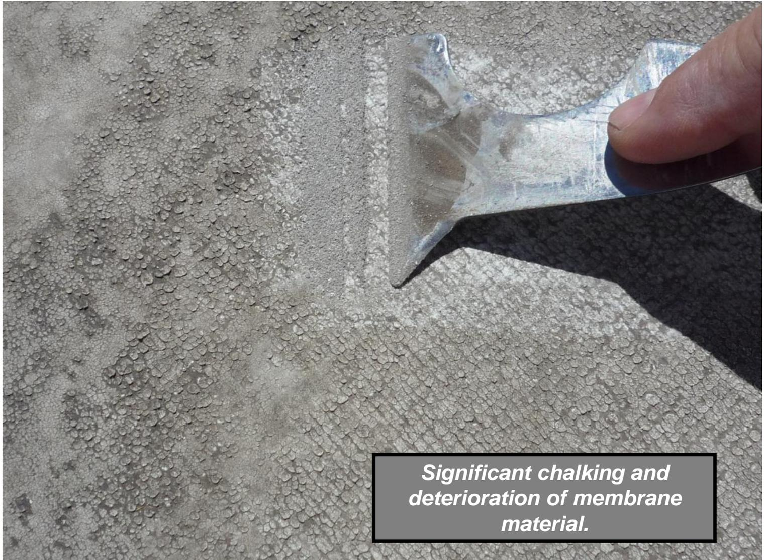
*Significant chalking and deterioration of membrane material.*
