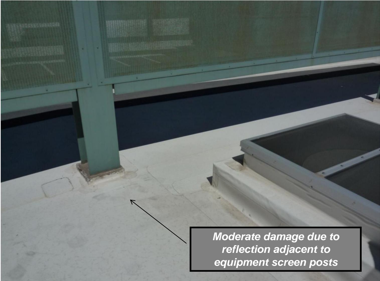
*Moderate damage due to reflection adjacent to equipment screen posts*
