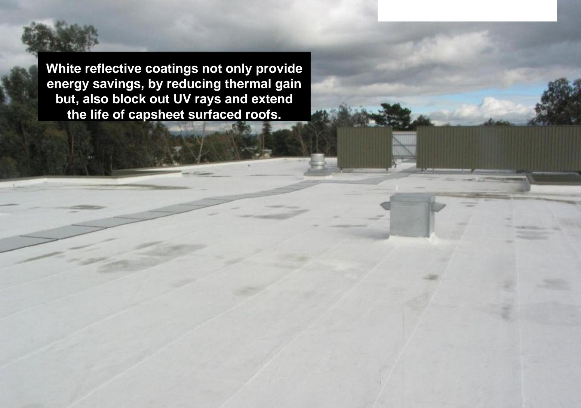
**White reflective coatings not only provide energy savings, by reducing thermal gain but, also block out UV rays and extend the life of capsheet surfaced roofs.**
