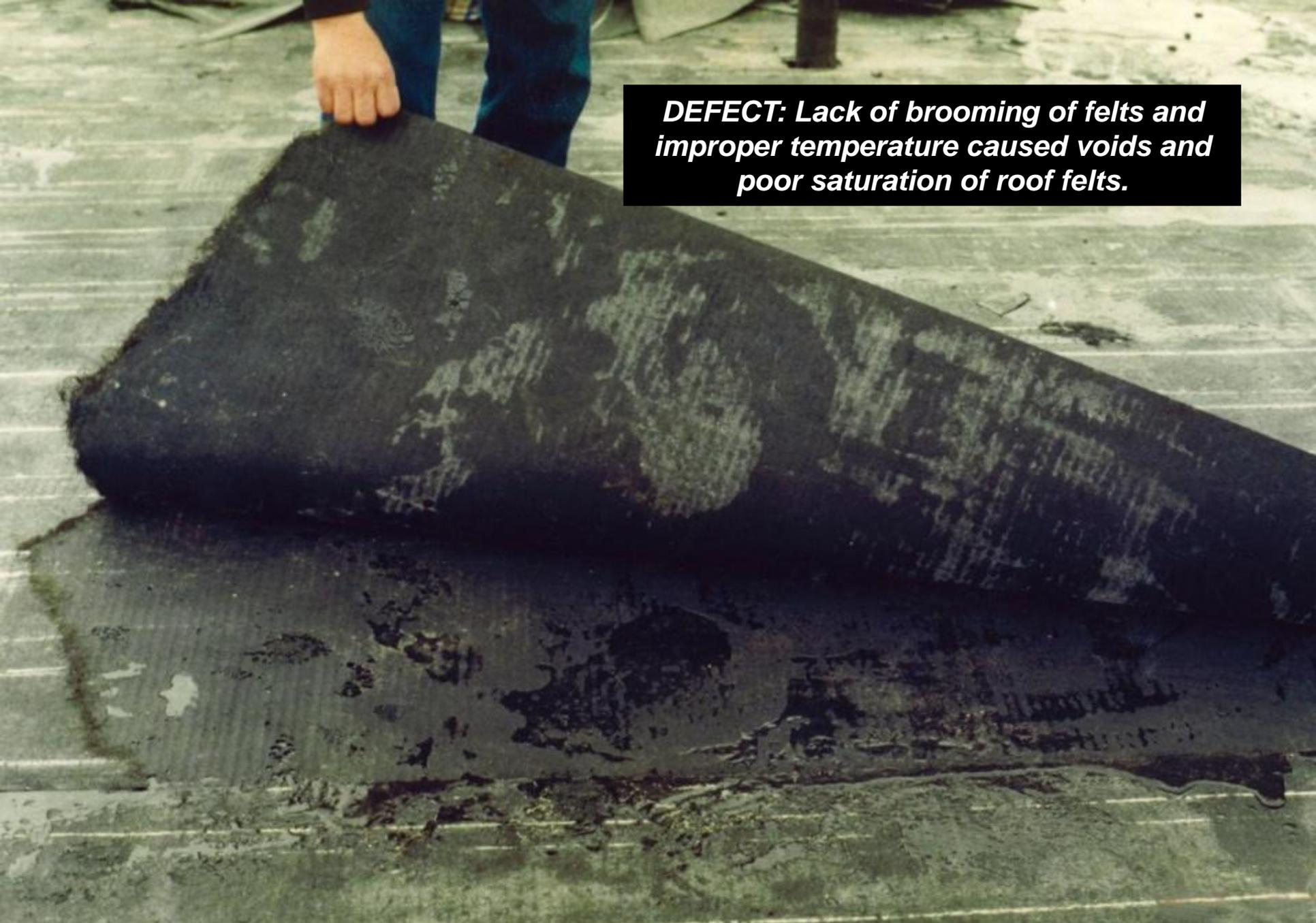
***DEFECT: Lack of brooming of felts and improper temperature caused voids and poor saturation of roof felts.***
