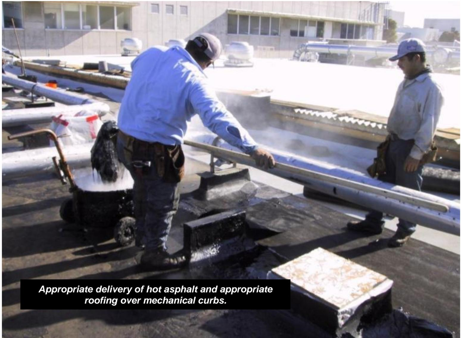
*Appropriate delivery of hot asphalt and appropriate roofing over mechanical curbs.*
