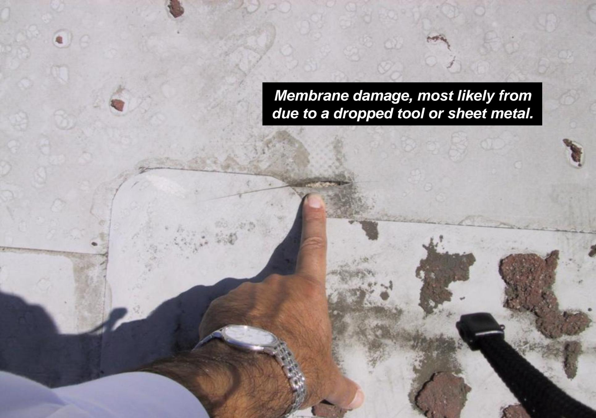
***Membrane damage, most likely from due to a dropped tool or sheet metal.***
