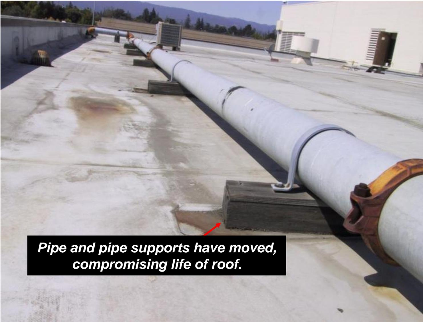
*Pipe and pipe supports have moved, compromising life of roof.*
