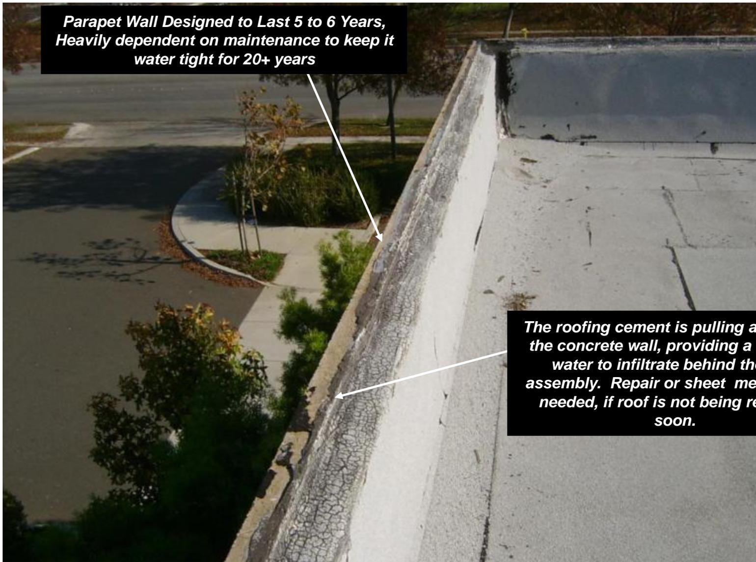
*The roofing cement is pulling away from the concrete wall, providing a route for water to infiltrate behind the roof assembly. Repair or sheet metal cap is needed, if roof is not being replaced soon.*
