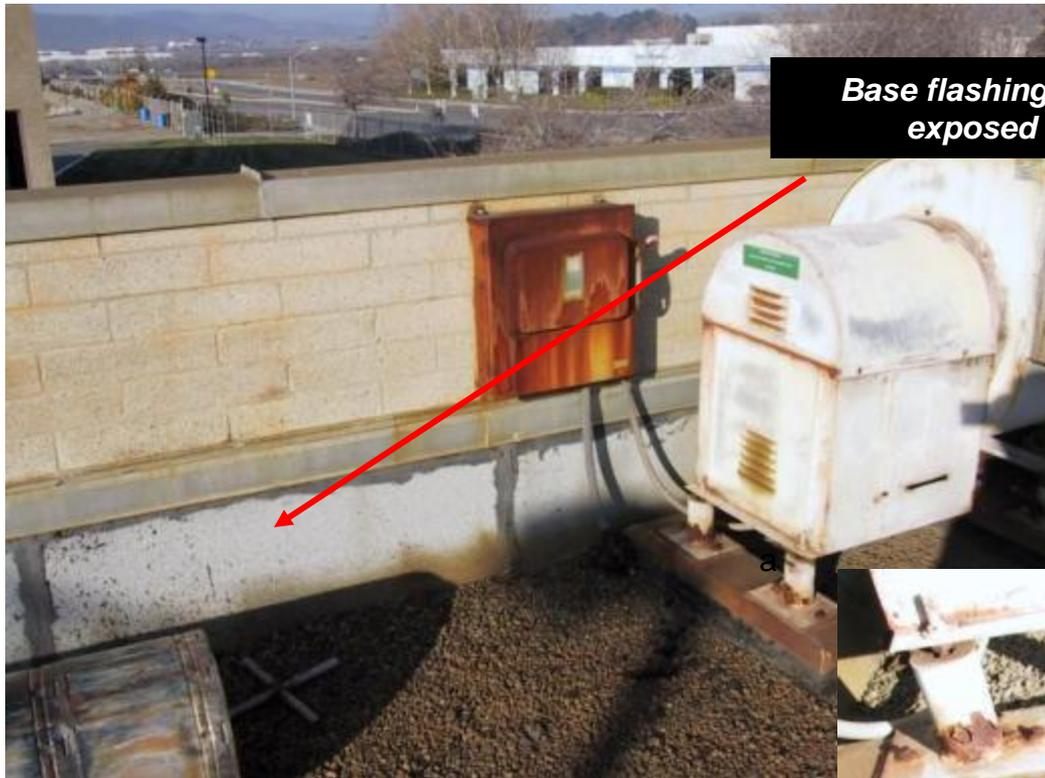
*Base flashings (Horizontal to vertical junction) are exposed to more UV and physical abuse.*
