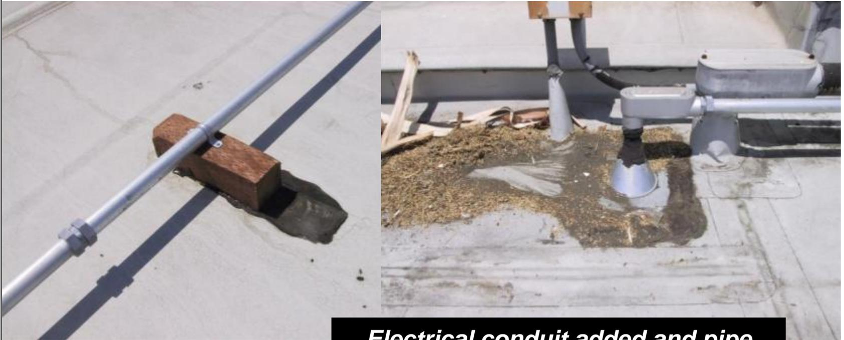
***Electrical conduit added and pipe jack added, both set in mastic that is incompatible with PVC.***
