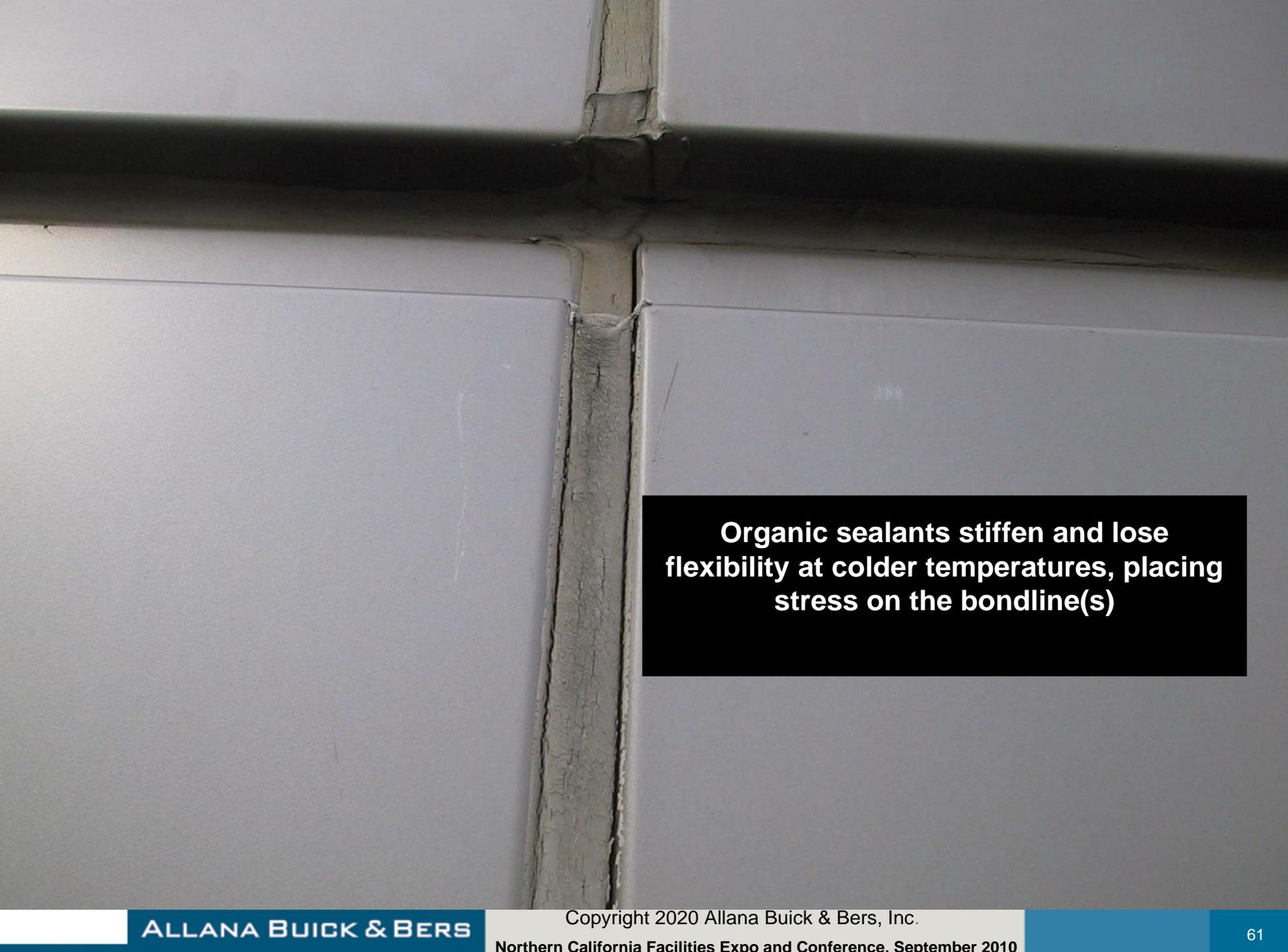
**Organic sealants stiffen and lose flexibility at colder temperatures, placing stress on the bondline(s)**
