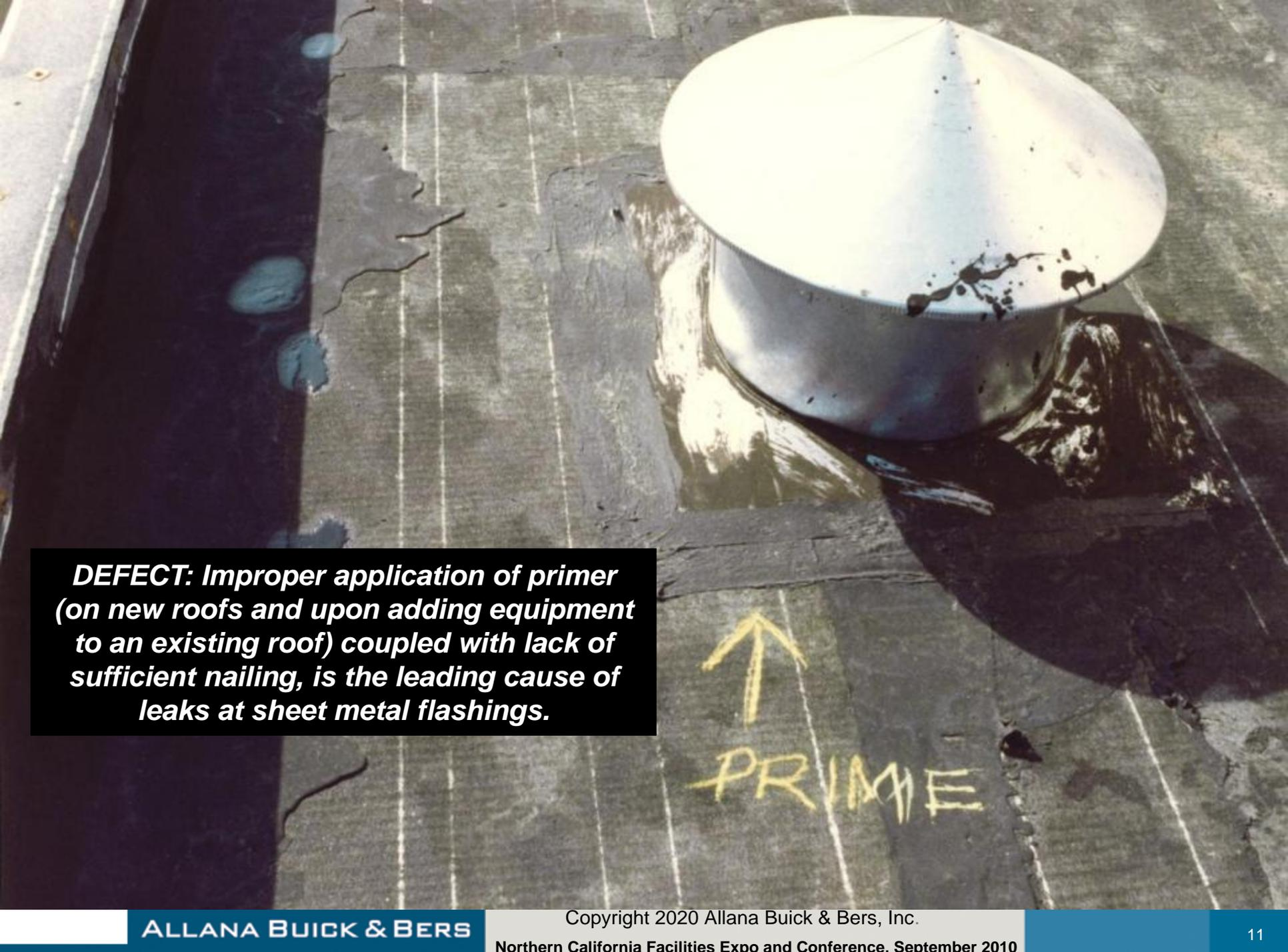
***DEFECT: Improper application of primer (on new roofs and upon adding equipment to an existing roof) coupled with lack of sufficient nailing, is the leading cause of leaks at sheet metal flashings.***
