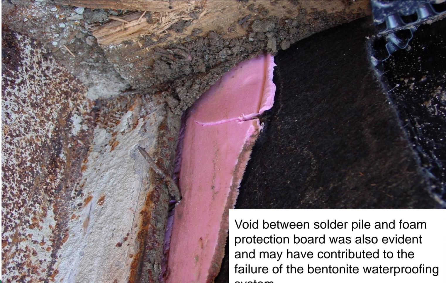
Void between solder pile and foam protection board was also evident and may have contributed to the failure of the bentonite waterproofing system.
