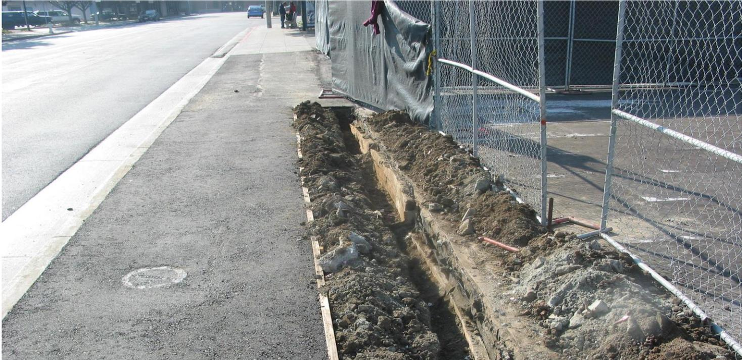
Excavation of the soil behind the wood lagging revealed that once the wood gets wet, it swells, bends and twists, especially if there are voids between the soil and wood.
