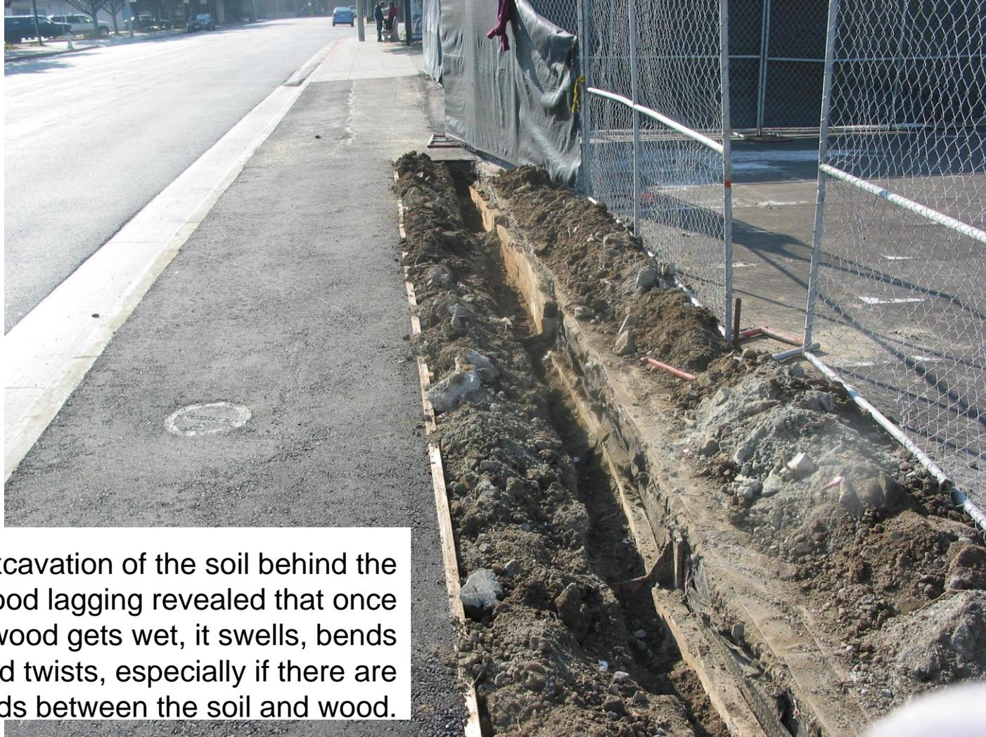
Excavation of the soil behind the wood lagging revealed that once the wood gets wet, it swells, bends and twists, especially if there are voids between the soil and wood.
