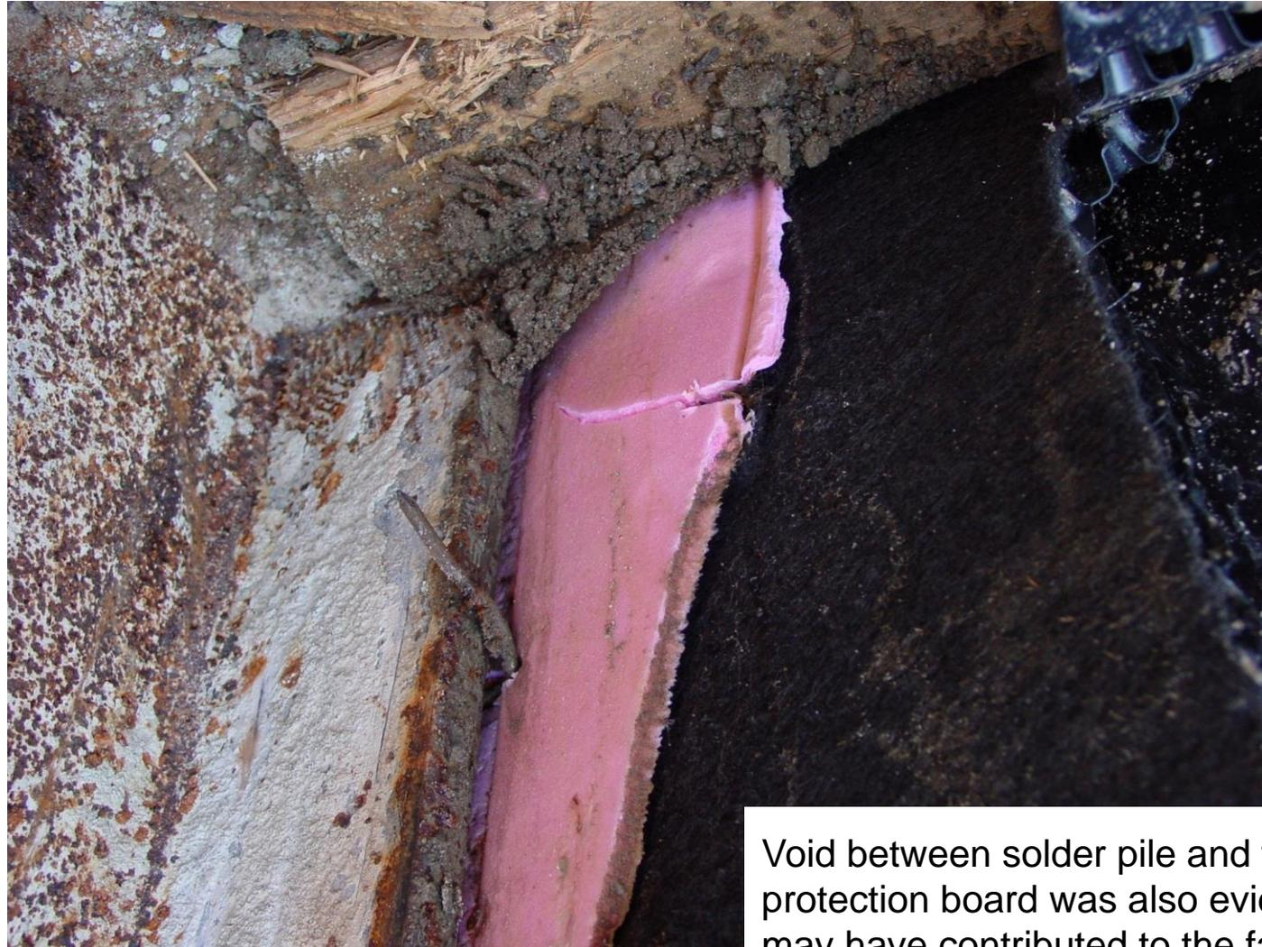
Void between solder pile and foam protection board was also evident and may have contributed to the failure of the bentonite waterproofing system.
