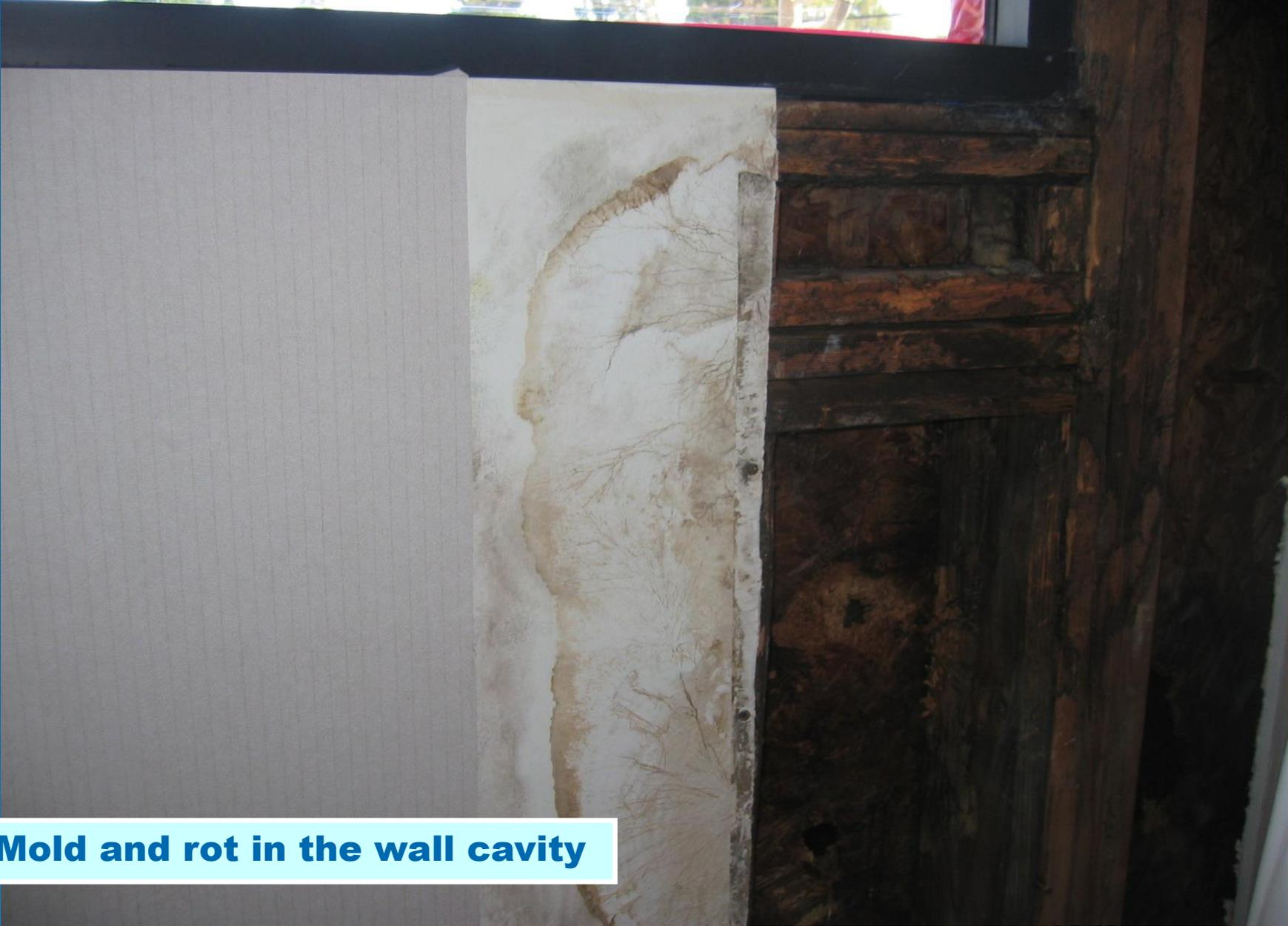
A photograph showing a cross-section of a wall. On the left is a smooth, light-colored surface. In the center, a vertical strip of material is peeling away, revealing a dark, textured interior. This interior shows significant mold growth and wood rot, with a large, irregular, brownish stain. To the right, dark wooden framing is visible. The overall scene illustrates the damage caused by moisture and mold in a wall cavity.
