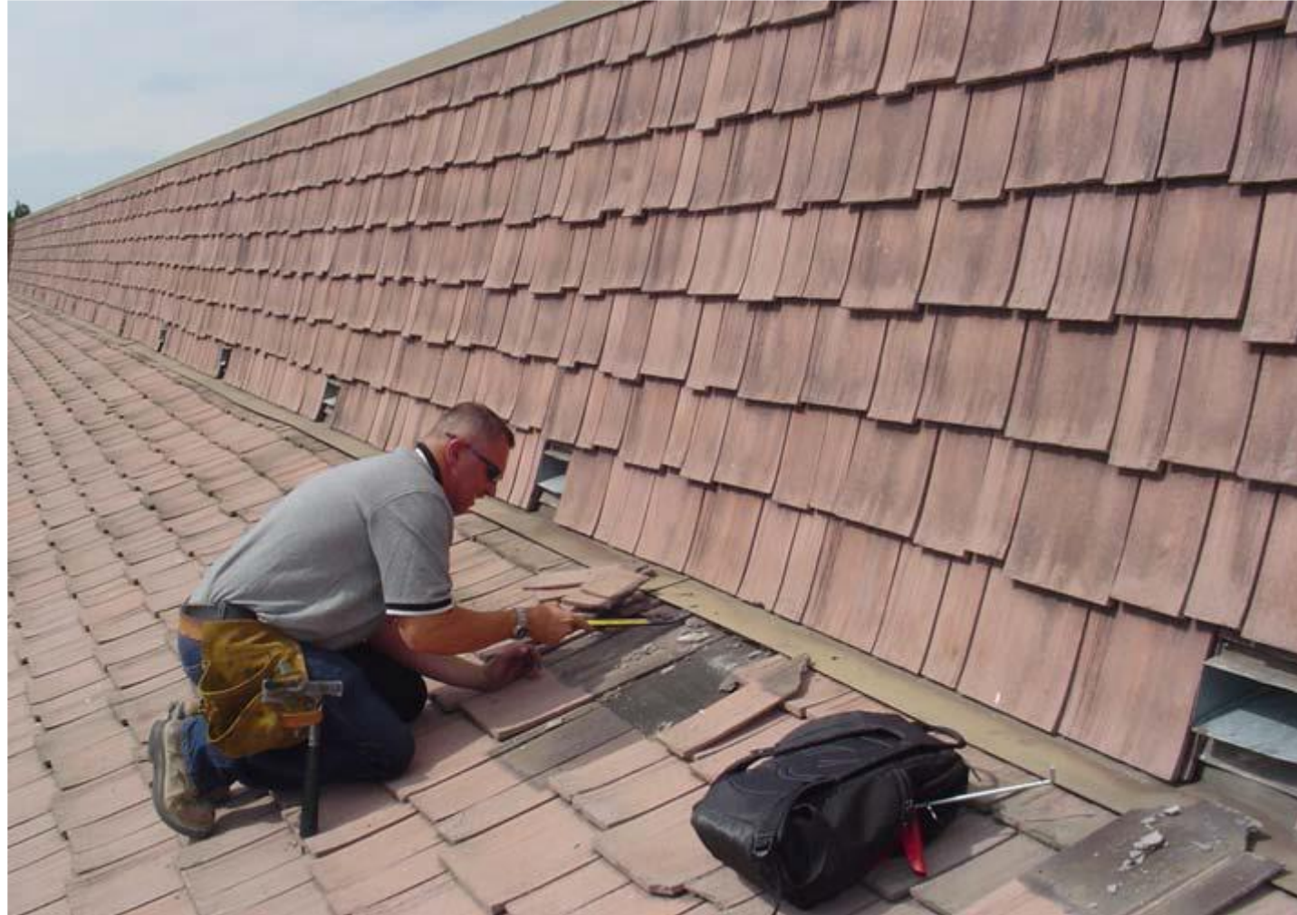
Testing occurred 3 – 5 years in service
