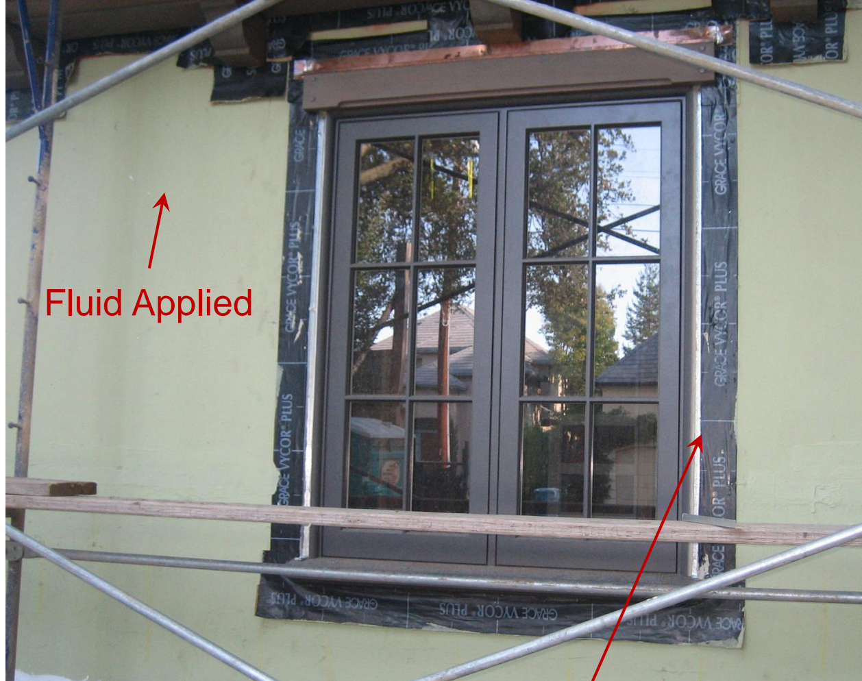
Window sealed with Flexible Flashings
