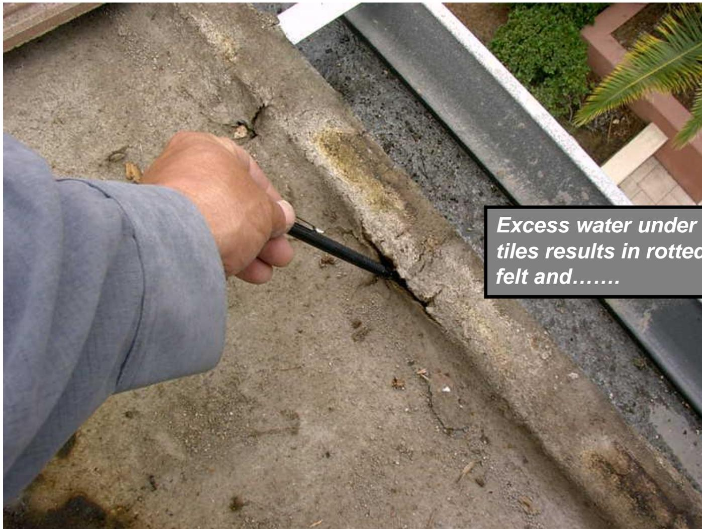
*Excess water under the tiles results in rotted felt and.....*
