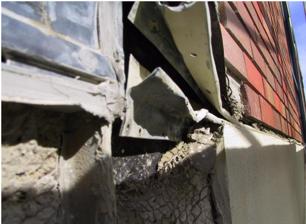
TOP: This 2 piece expansion joint has a very small overlap between the top and bottom piece. Wind driven rain can direct water behind the joint. BOTTOM: Exploded view of the two-piece expansion screed.
