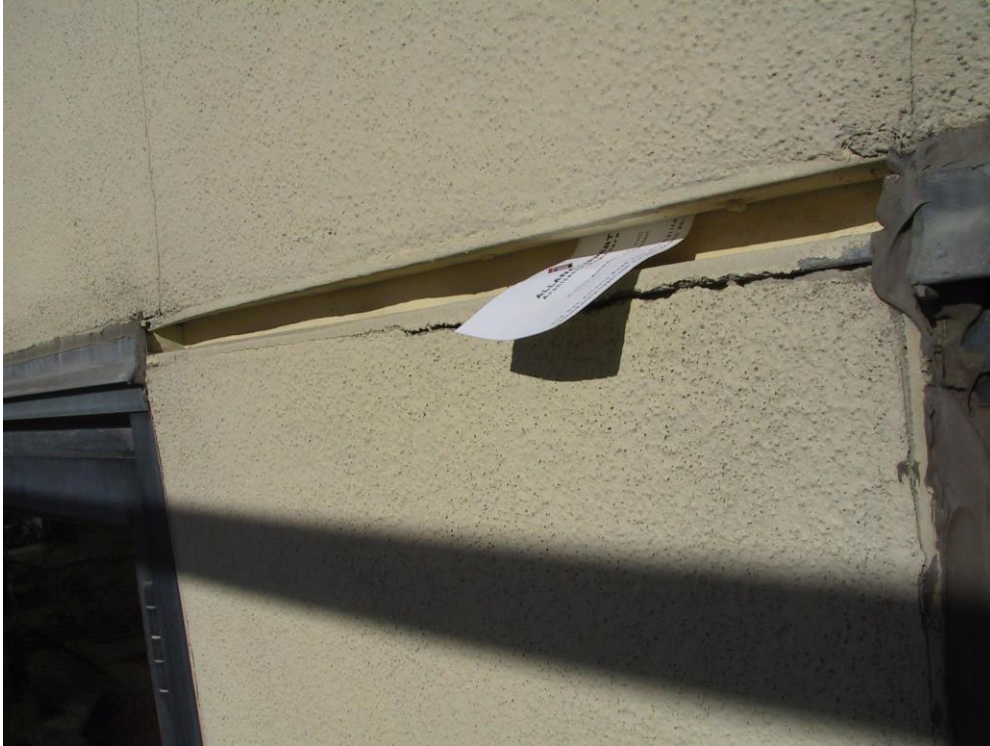
TOP: This 2 piece expansion joint has a very small overlap between the top and bottom piece. Wind driven rain can direct water behind the joint. BOTTOM: Exploded view of the two-piece expansion screed.
