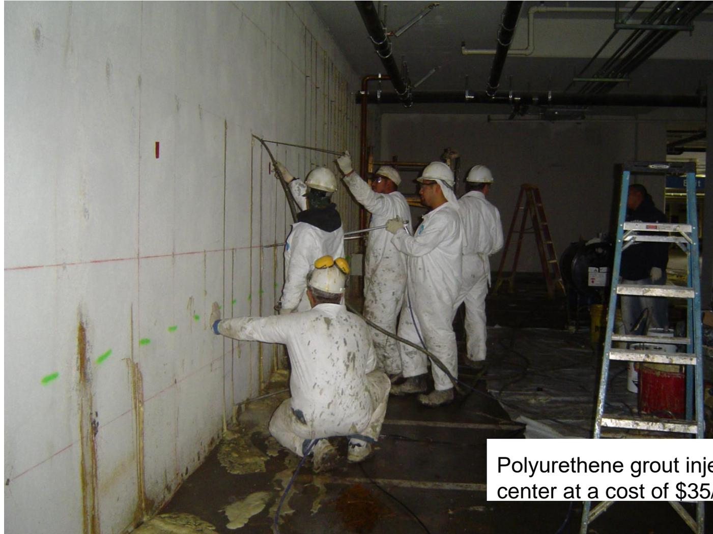
Polyurethane grout injection 2' on center at a cost of \$35/SF
